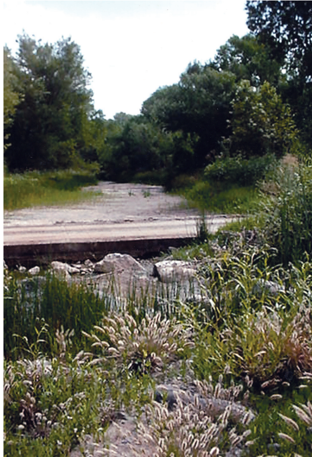
Figure A47. Looking upstream at ford and Agua Fria channel. Fish can move across the ford only when it is submerged.
