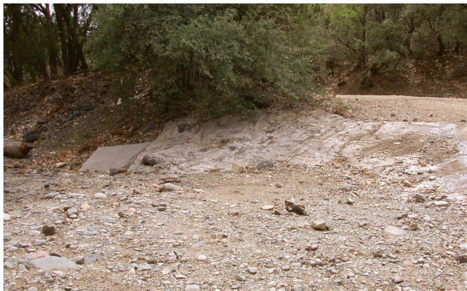
Figure A51. Concrete apron and grouted riprap prevent downstream scour and scour around edges of the ford.
