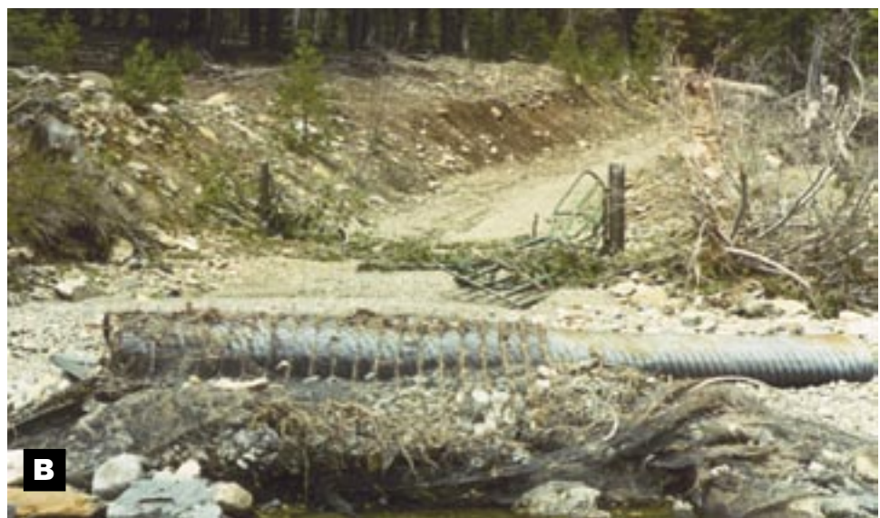
Figures A74a and b. The original gabion vented ford. (a) as built and (b) after the 1986 storm.
