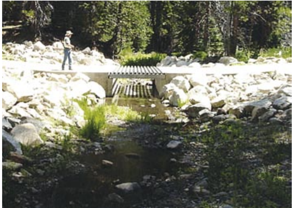
Figure A80. One of several grating-top box culvert fords on tributaries of the North Fork Consumnes River.
