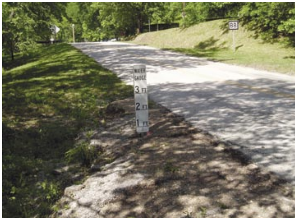
Figure 4.22—Typical depth marker, Missouri county road.
