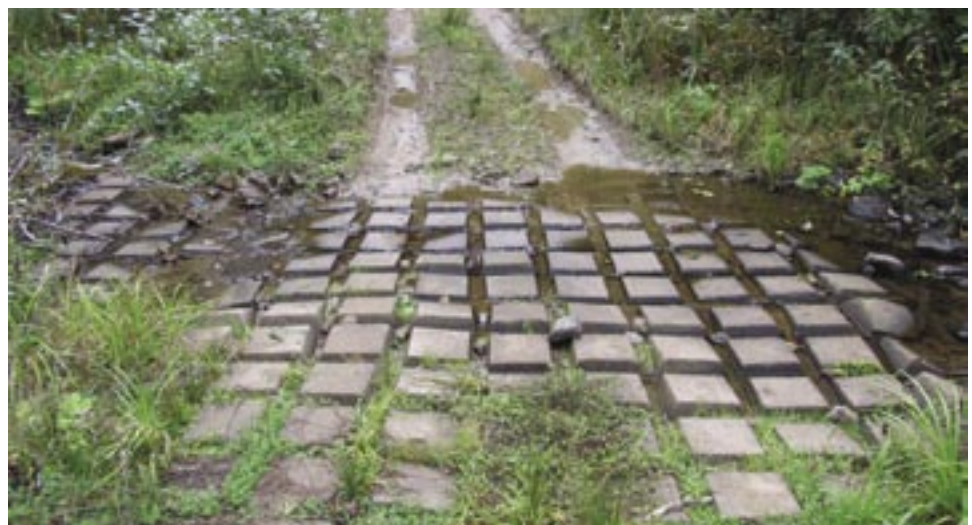
Figure A31. The ford permits low flow passage for aquatic species even though the blocks have settled unevenly.
