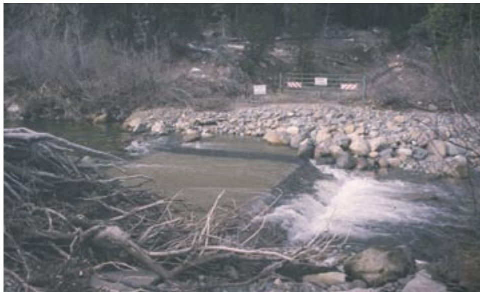
Figure A78. After a major storm, medium and large boulders and large root wads cover the ford, but the structure is undamaged.
