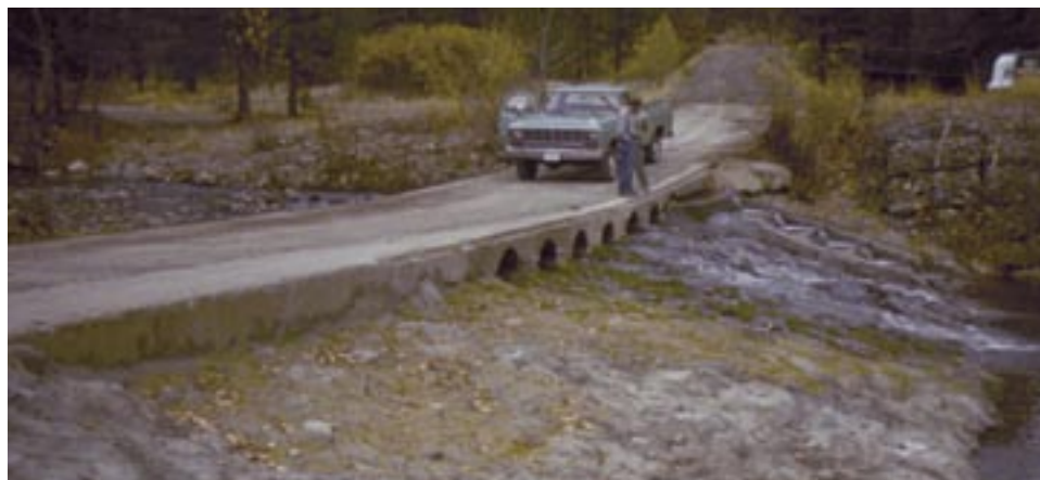
Figure A98. Moonlight Crossing prior to the 1997 flood. Note the weakly grouted small riprap armoring the downstream apron. There is no cutoff wall.
