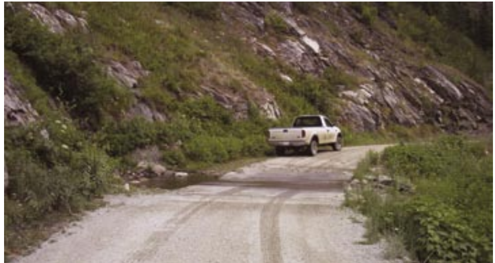
Figure A60. Ford is located on a valley bottom road at the base of an avalanche chute.
