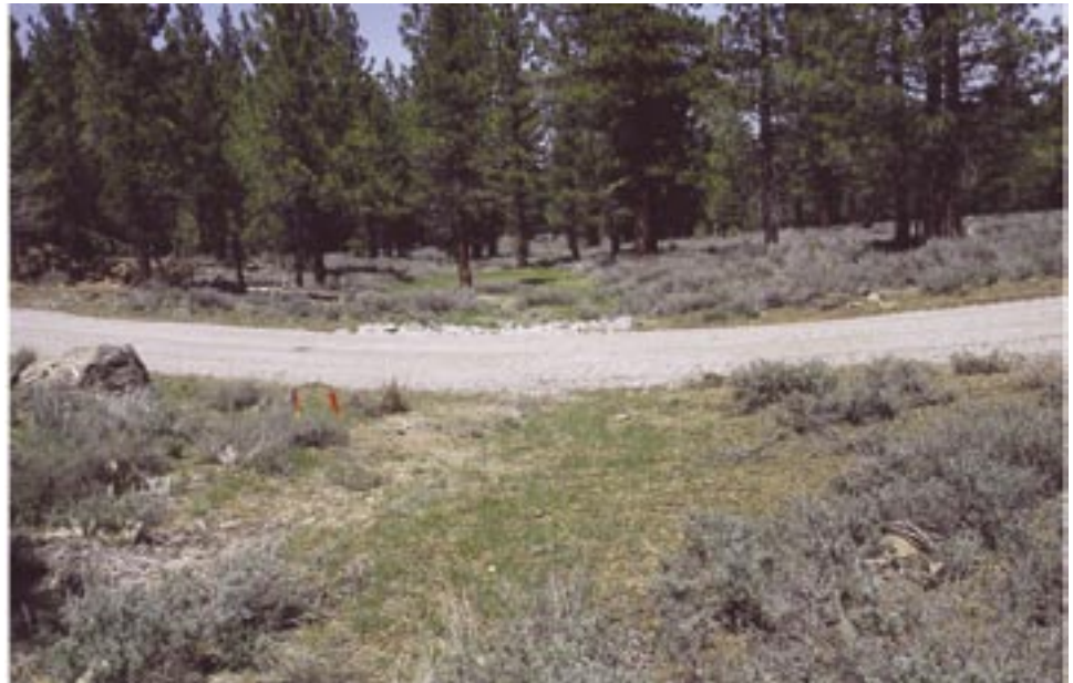
Figure 5.2—At-grade improved rock ford, Plumas National Forest.
