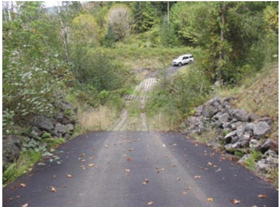
Figure A27. Fitzpatrick cable concrete mat ford.
