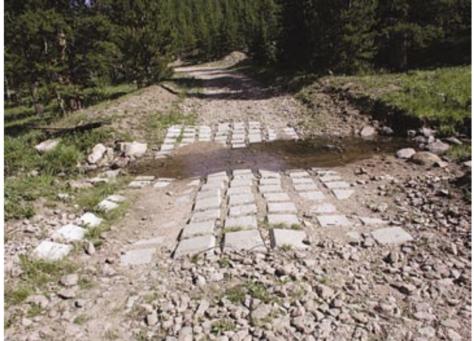
Figure 5.6—Cable concrete block ford, Bighorn National Forest, Wyoming. Note that mat should extend higher to protect the crossing adequately.
