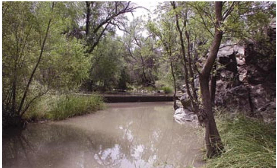
Figure 5.4—Concrete slab creates fish barrier at low flow, Seven Springs, Tonto National Forest.
