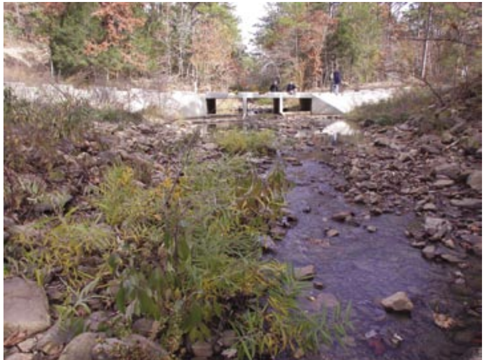
Figure A86. Looking upstream at the concrete vented ford and splash apron.
