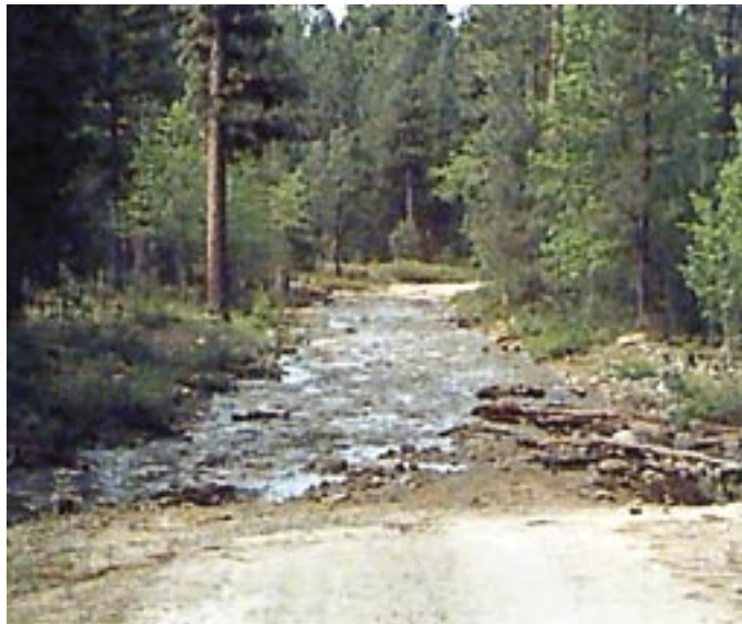
Figure A7—Plugged culvert causes water diversion down road before construction of rock fords.
