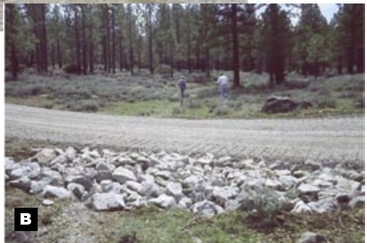
Figures A1a and A1b. Red Clover rocked dip. Figure A1a. Flow is from left to right across the dip. Figure A1b. View is upstream.
