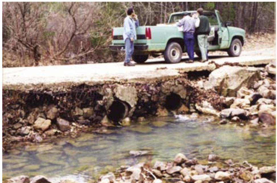
Figure A87. The previous crossing on road 887 at Rocky Creek was a gabion-culvert structure that was frequently damaged during high flows.
