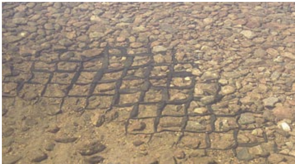
Figure A39. GEOWEB exposed, probably by tire action.
