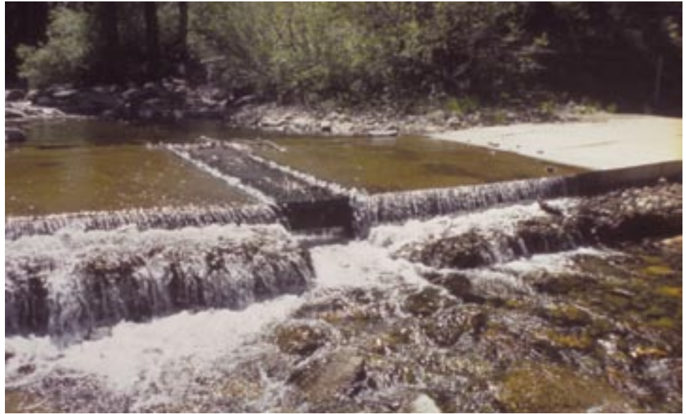
Figure A79. Grubbs ford immediately after construction in 1986. The vent appears to be a velocity barrier when it is not plugged.
