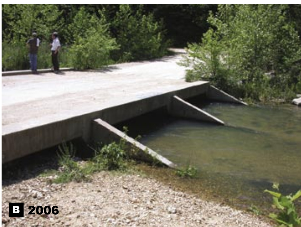
Figures A124a and A124b. Downstream side of the box culvert crossing. Between 2003 and 2006, gravel bar enlarged to block one box.
