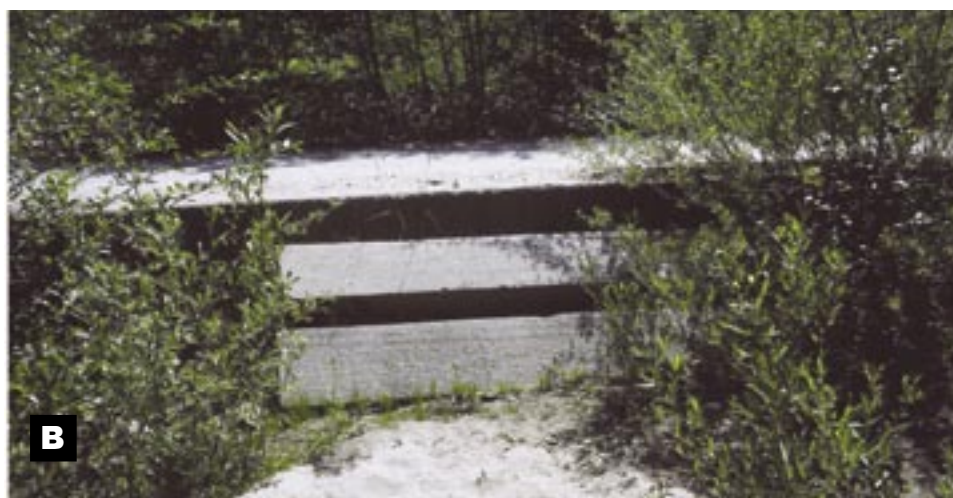
Figures A118a and A118b. Scour protection measures a) using riprap with vegetation along the channel (left) and b) concrete blocks and gabions along the elevated roadway (right).
