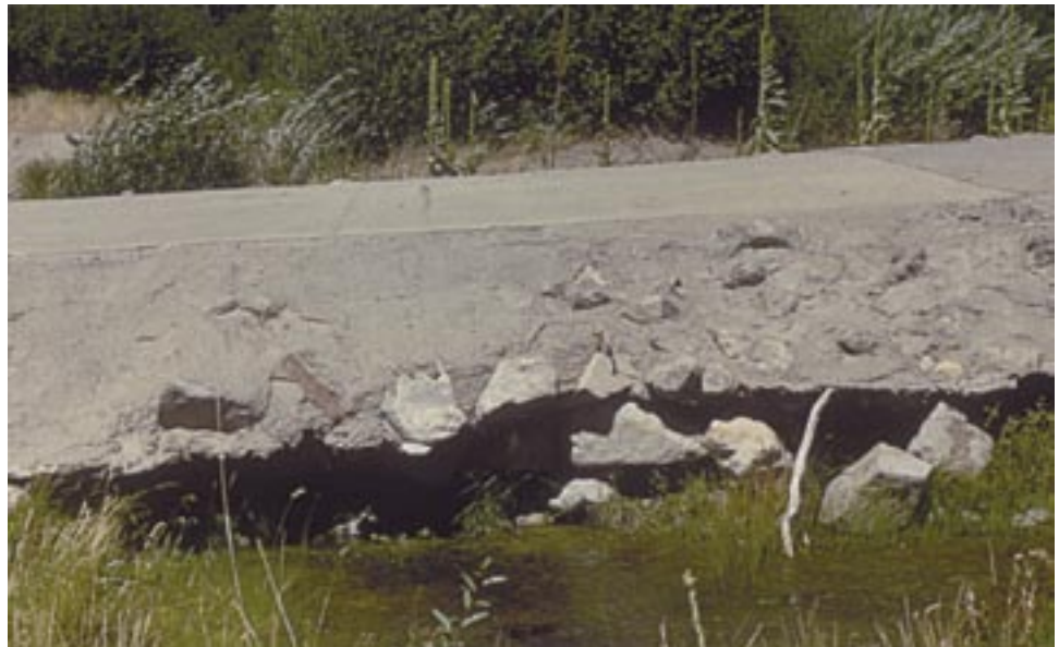
Figure A65. Downstream scour under the slab after the 1982 flood. The repair was to add a 5-foot-deep vertical concrete cutoff wall.
