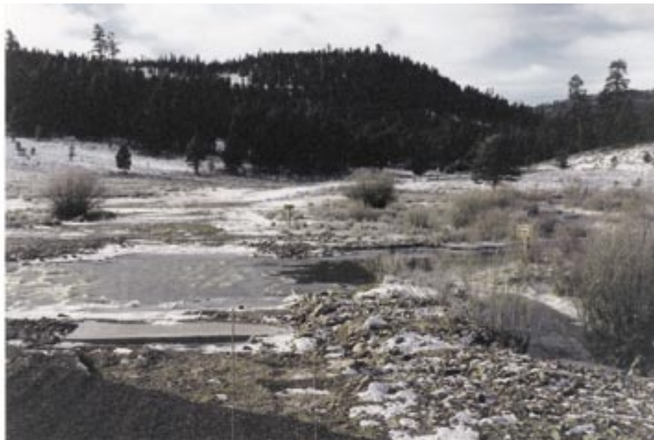
Figure A59. Shortly after the 1997 New Year's Day flood. Some gravel washed from the approaches (in foreground) was the only damage from the largest flood on record.
