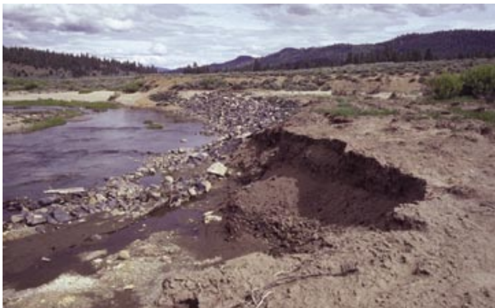
Figure 4.16—Looking downstream at a failed riprap installation on Red Clover Creek, Plumas National Forest.
