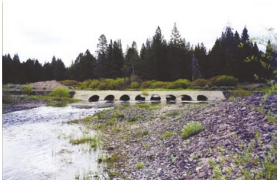
Figure 5.13a—Murdock vented ford, Plumas National Forest, California looking upstream (note excavated sediment upstream of ford).
