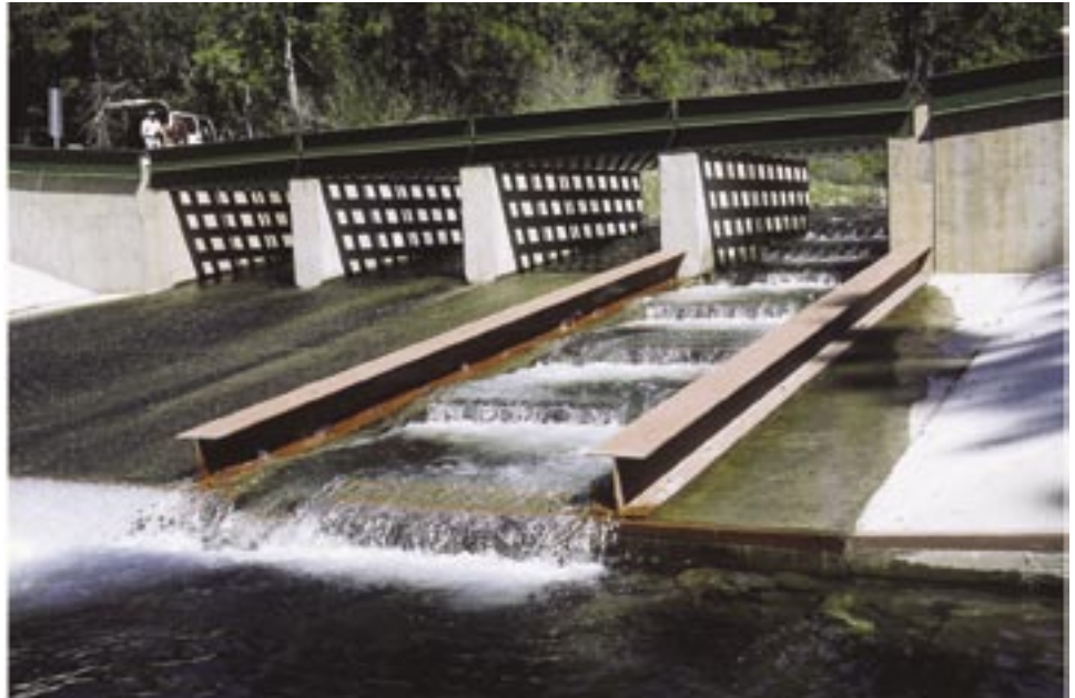
Figure A102. Detail of the fish ladder built into the Moonlight Crossing.
