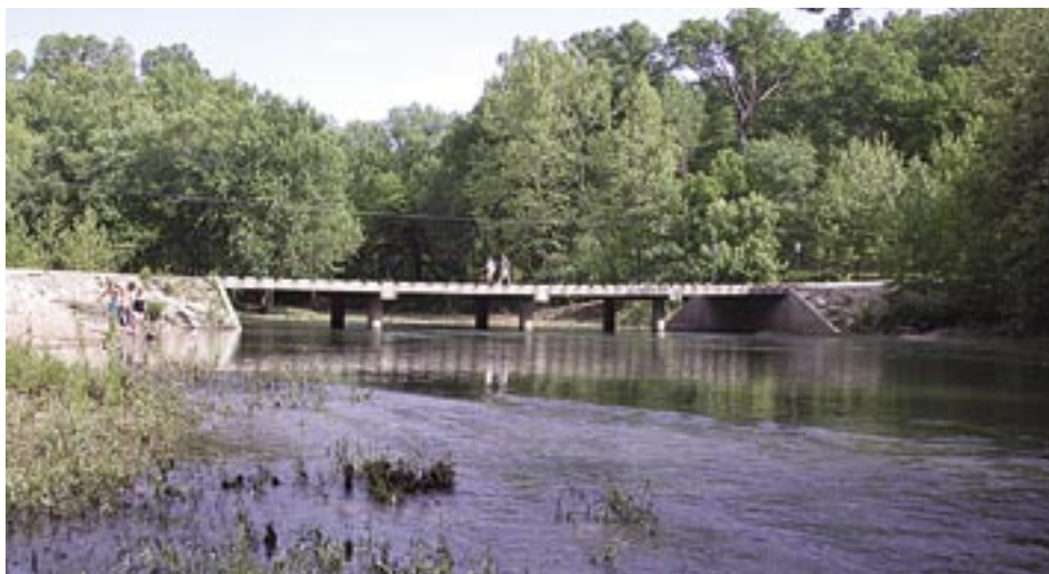
Figure 1.8—Low-water bridge at Boiling Springs, Big Piney River, Missouri.
