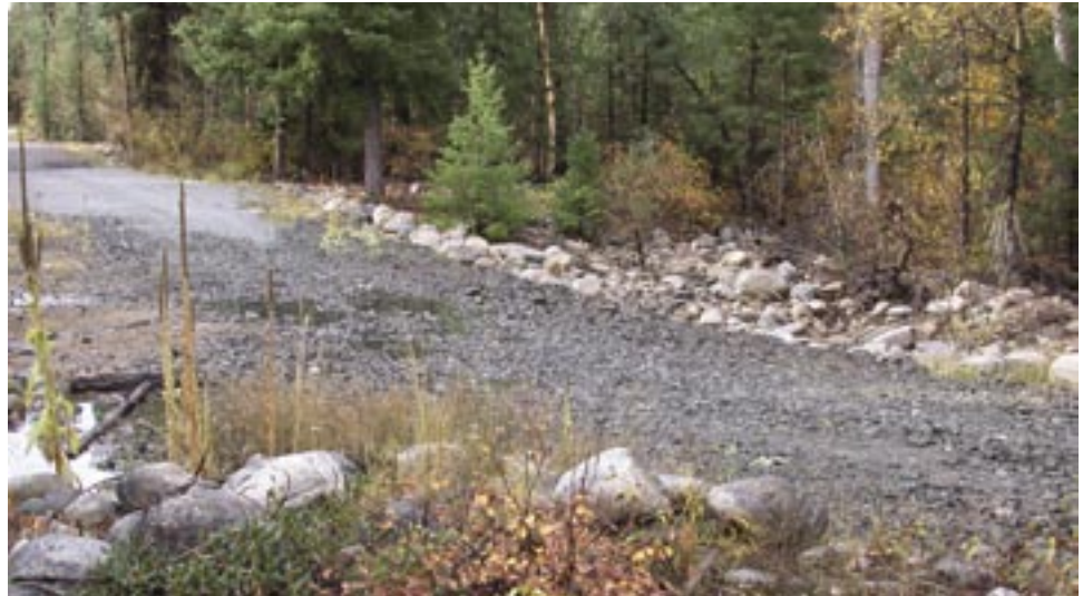
Figure A10. Hardened dip on East Chewuch Road.
