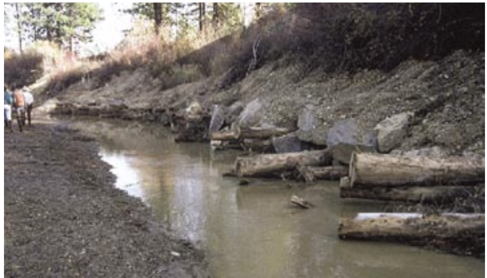
Figure 4.18—Rootwads and boulders used to stabilize a high streambank, Wolf Creek restoration project, Greenville, California, 1990.
