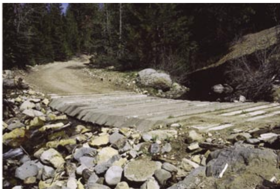
Figure A22. Willow Creek concrete plank ford.
