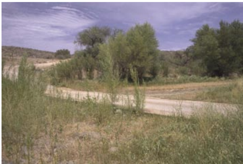
Figure A44. Oblique view of ford and aggraded upstream channel.
