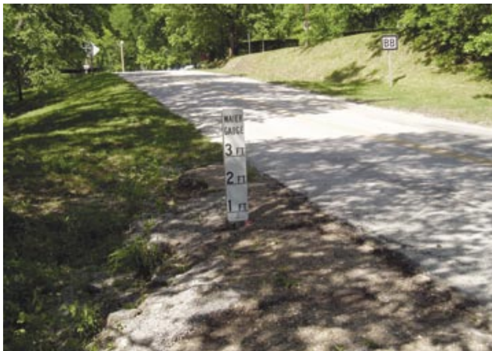
Figure 4.22—Typical depth marker, Missouri county road.
