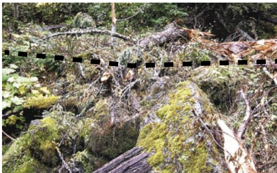
Figure A13. Stable, moss-covered rocks on the splash apron with pieces of fallen snag. Dashed line indicates approximate road surface.
