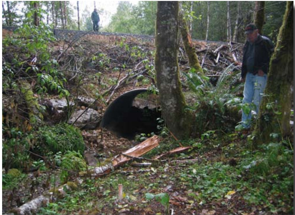
Figure 7.11—Clearing debris scattered for erosion control.
