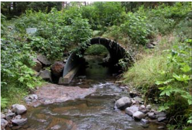
Figure 7.4—1-piece open-bottom arch.
