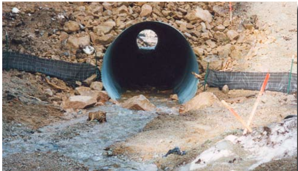
Figure 7.22—Typical silt-fence installation.
