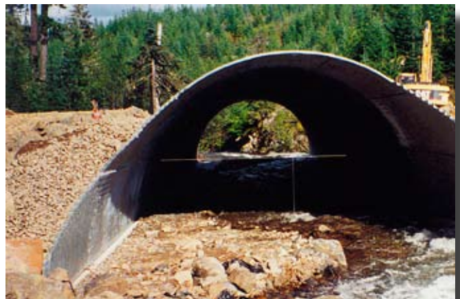
Figure 7.5—Multiplate open-bottom pipe arch.
