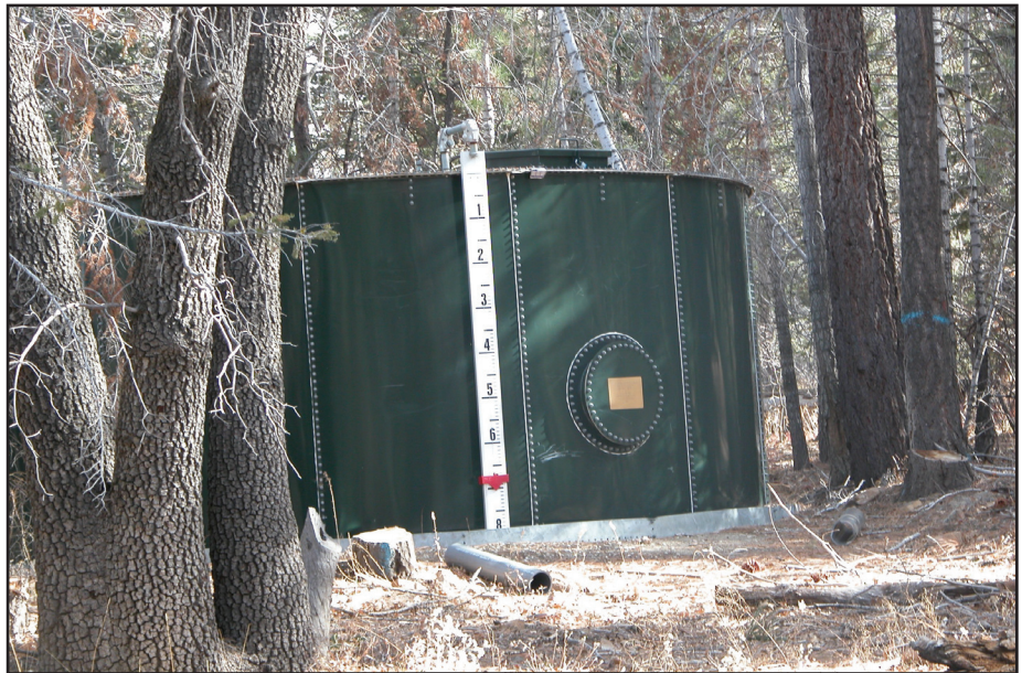
Figure 27—Aboveground tank located outside of riparian area.
