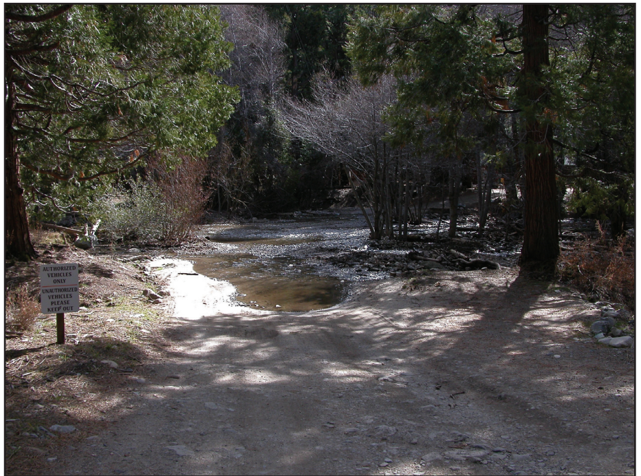
Figure 18—Site is not well armored to prevent erosion and sediment delivery.
