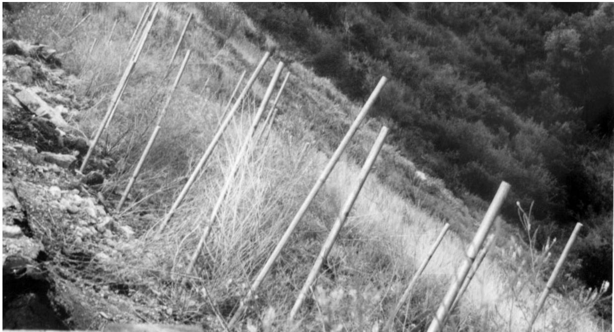
Photo 14. Three rows of launched soil nails in the slope in photo 13 before cut-off of the nails.
