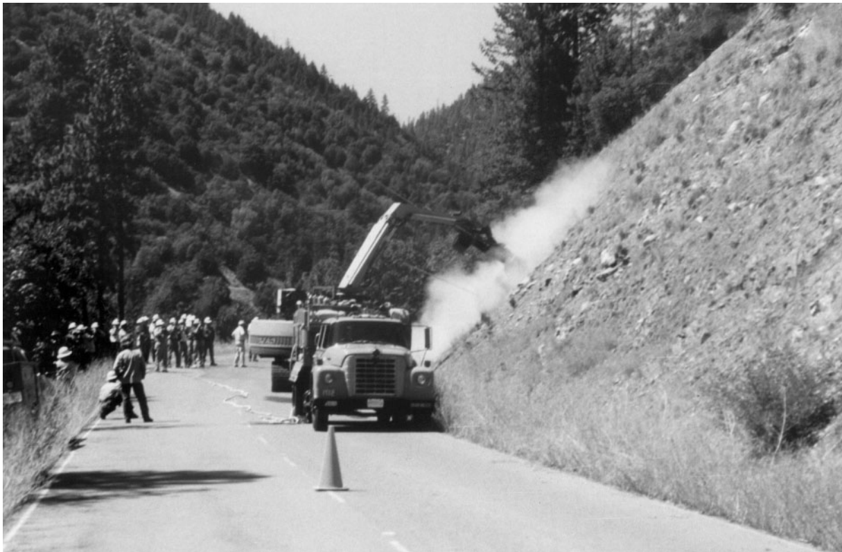
Photo 18. Launching a soil nail into a cutslope on the Klamath NF in Northern California.
