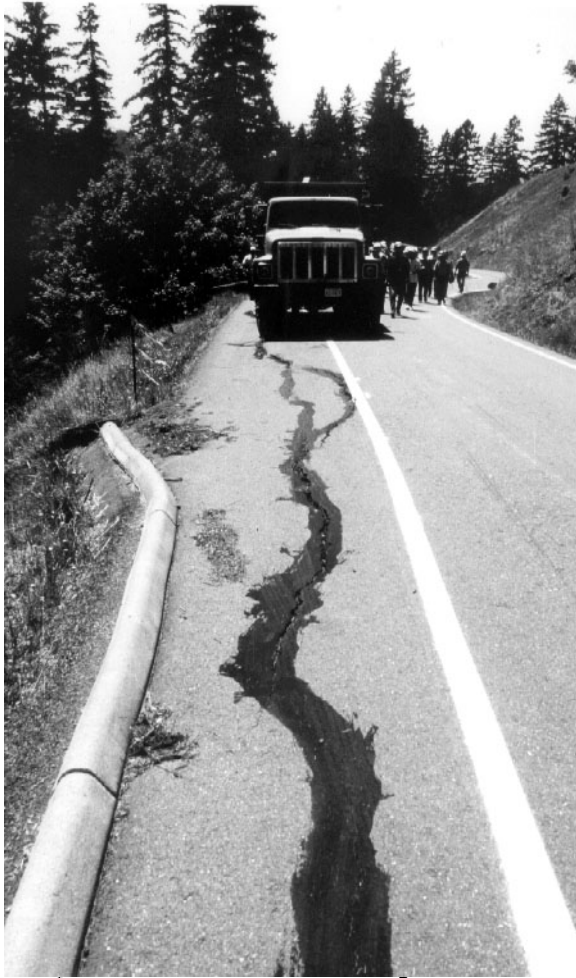
Photo 12. Showing the launch of a soil nail to retain the road shoulder and halt further crack development. Note the retention of vegetation on the site.
