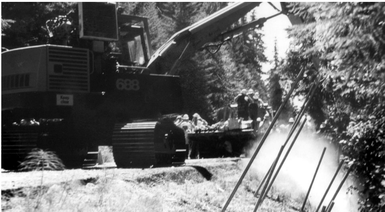
Photo 16. Launching a nail in the site in photo 15. Note the thickness of asphalt concrete pavement, indicating repeated patching of the pavement surface due to slope movement. Nails were cut off at the ground surface after the photo was taken.
