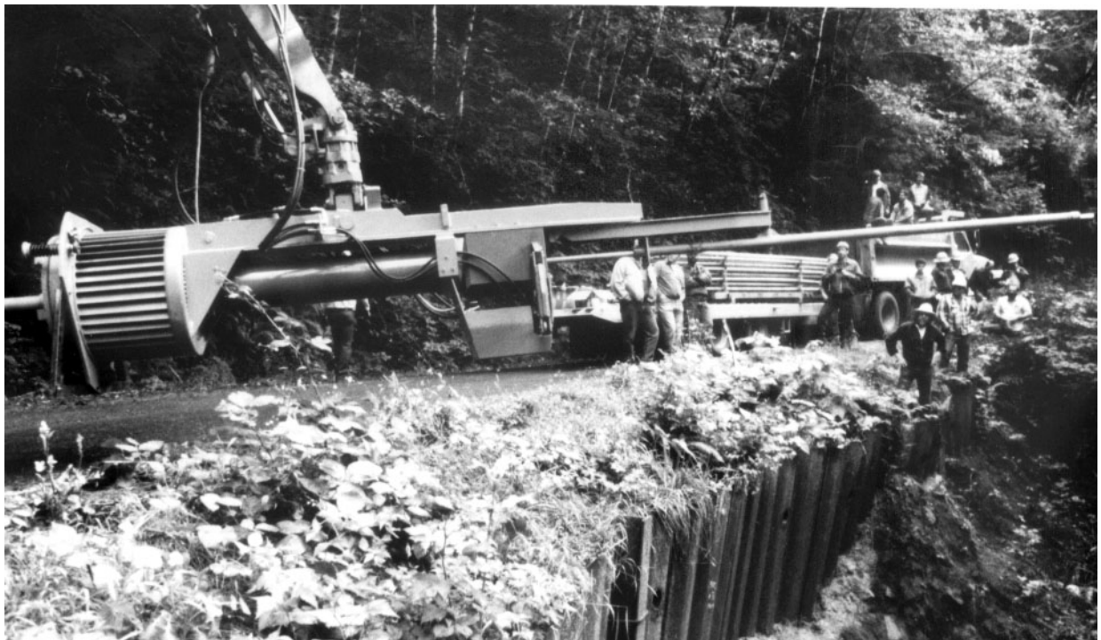
Photo 21. Positioning the launcher for installation of the soil nails.
