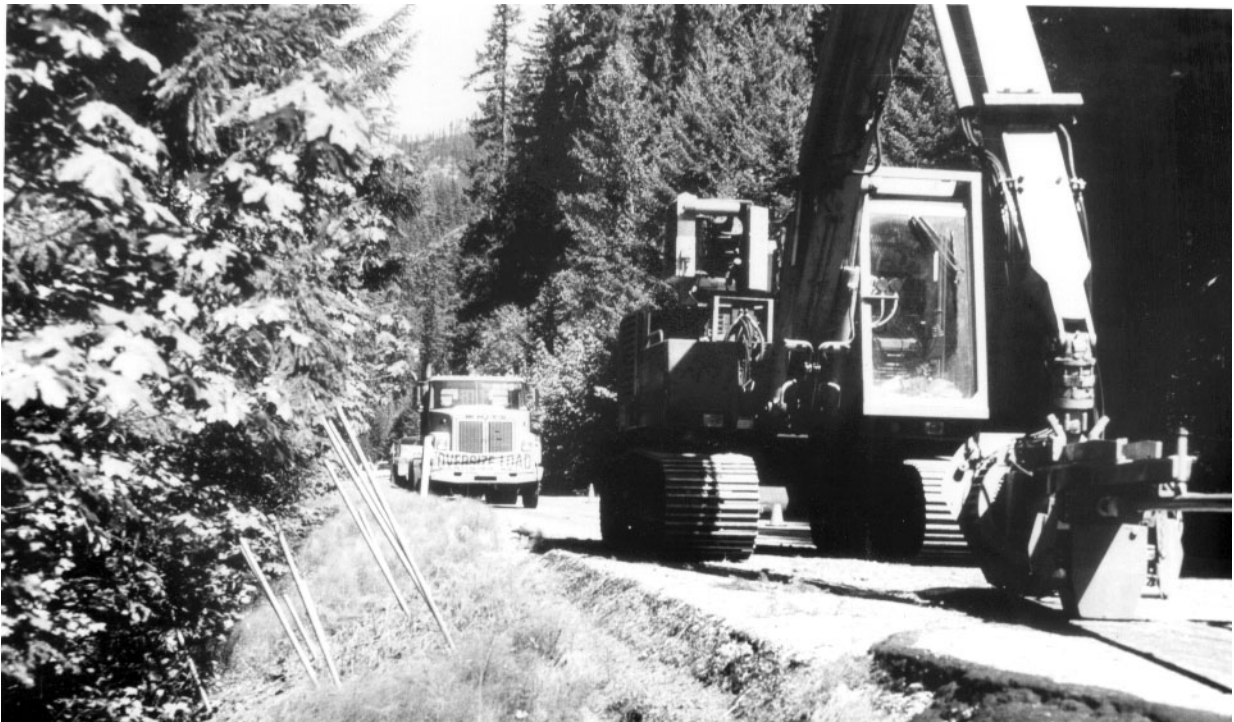
Photo 15. Excavator, launcher, and transport vehicle adjacent to installed nails. Note three rows of nails installed without disturbing the vegetation.
