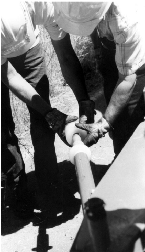
Photo 7. (above) Showing the barbed point of the soil nail for the lead transfer from the collet to the nail.
