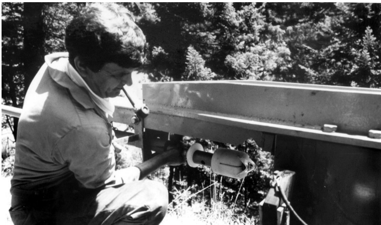
Photo 10. Soil nail in the support tube ready for placement of the collet and nail tip into the breech assembly.
