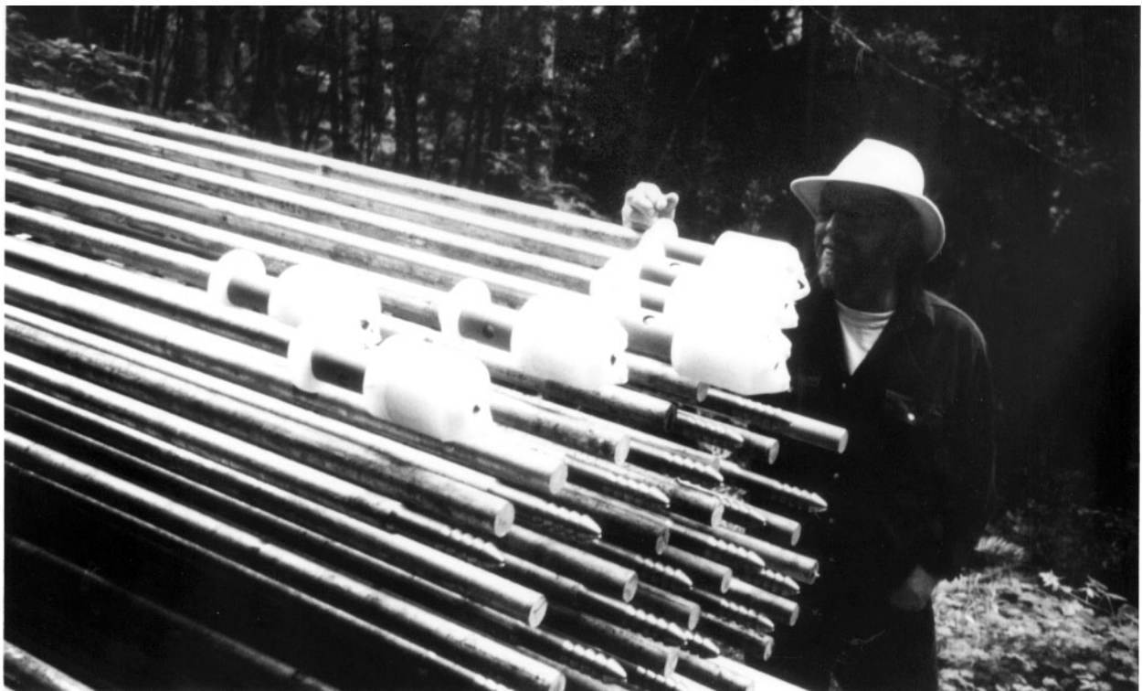
Photo 9. Soil nails on support trailer with some collets installed in preparation for launching.
