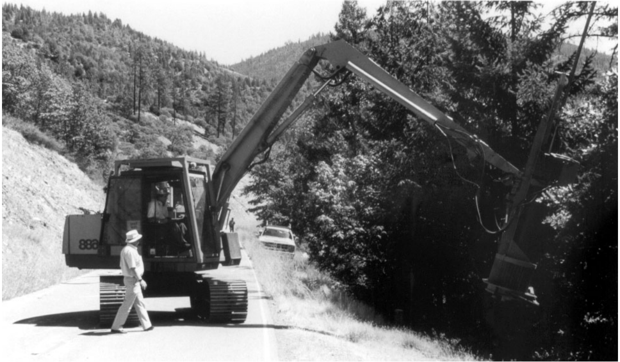
Photo 17. Positioning the soil nail launcher without removing roadside vegetation.
