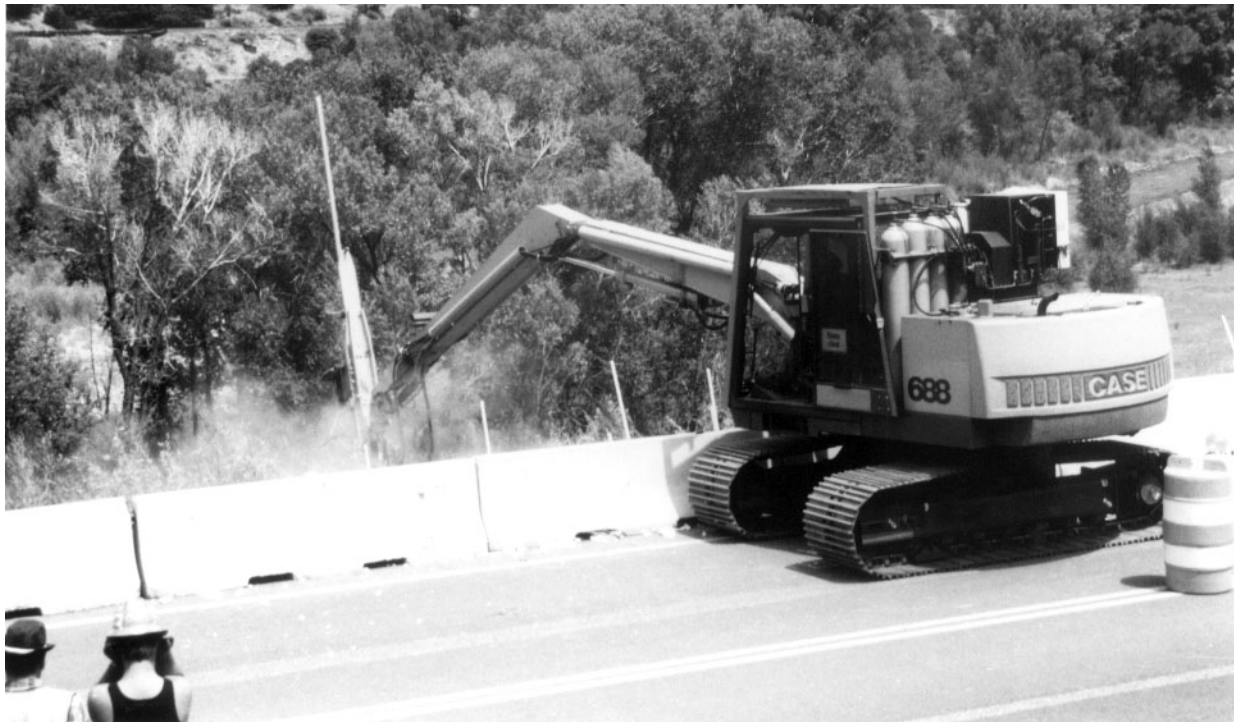
Photo 13. Reaching over a temporary guardrail to nail a failing slope in Colorado.
