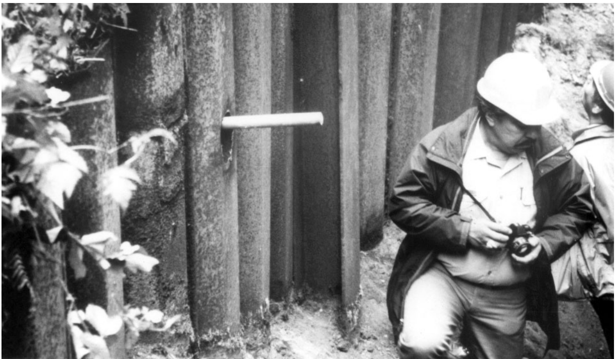
Photo 23. About 1.5 feet (0.5M) of the 18-foot (4.5 M) soil nail launched into the retaining wall backfill.
