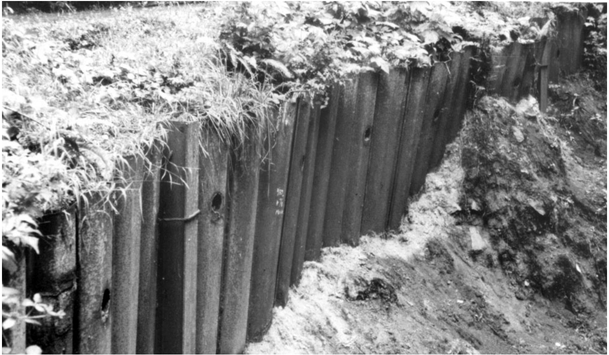
Photo 20. A driven sheet pile 1H-pile retaining wall in Oregon. Note the holes burned into the sheet pile for the launched soil nails.
