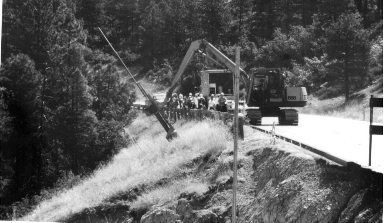
Photo 19. Ready to launch a soil nail into a failing slope in Colorado. The soil nails will prevent extensive downslope movement seen in the foreground.
