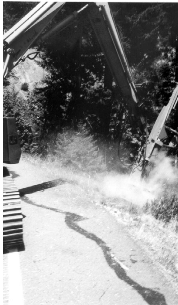
Photo 12. Showing the launch of a soil nail to retain the road shoulder and halt further crack development. Note the retention of vegetation on the site.
