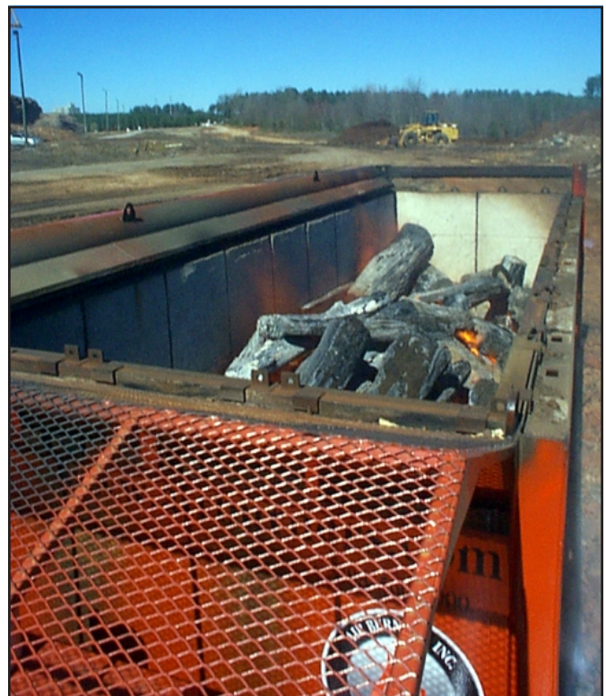
Figure 1—ACD in full operation (no visible smoke).
