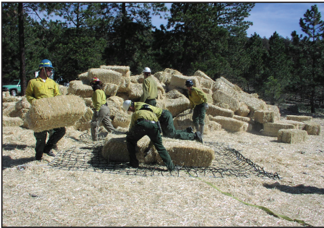
Figure 3—Rodeo method, retrieval line is stretched out under net.
