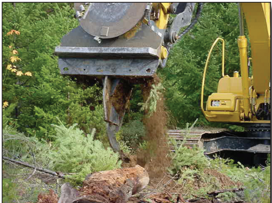
Figure 7-30—Subsoiling skid trail with a ripper shank on an excavator.
