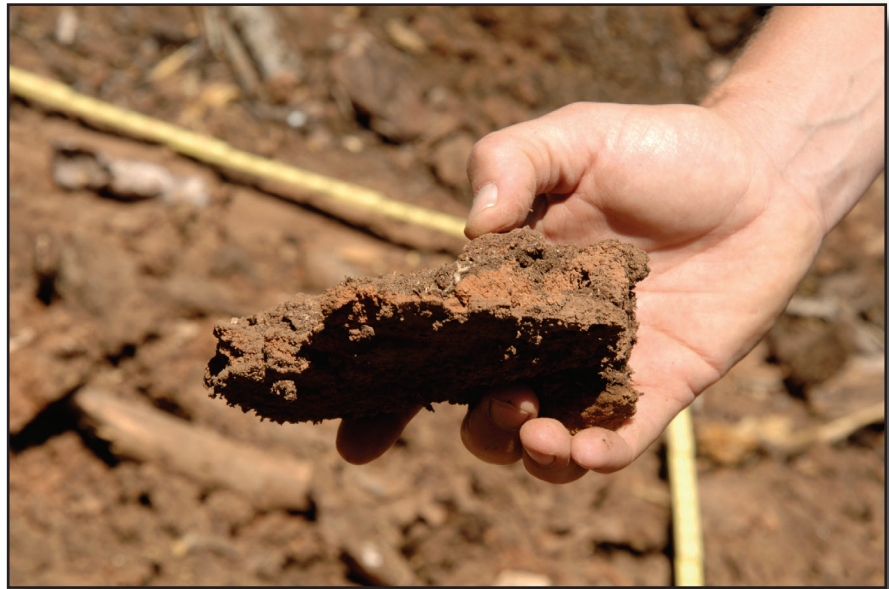
Figure 5-20—Compacted soil found within skid trail.
