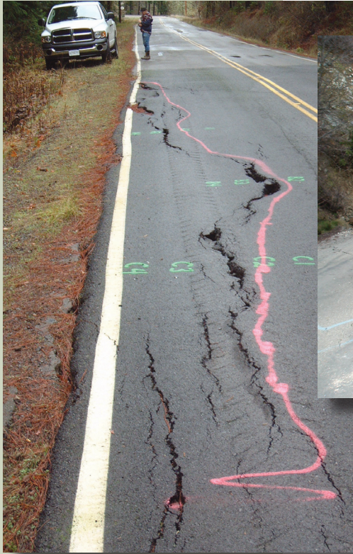
Figure 1—Cracking and settlement along top of slide in asphalt road, Region 6.
