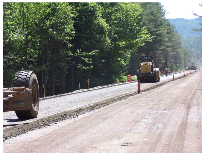
Figure 2.1c— Compacting (Charles Miller, Porter, Maine).
