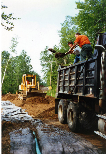
Figure 3.1h—Geosynthetic used for separation, White Mountain NF.
