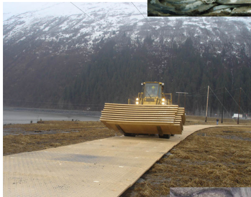
Figure 3.4d—Dura-Base road construction, Alaska. (Dennis Swarthout, Carol Huber).
