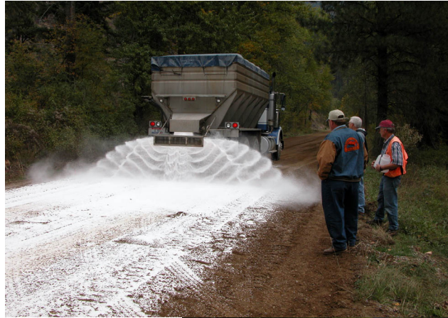
Figure 2.2a—Dry chloride application.
