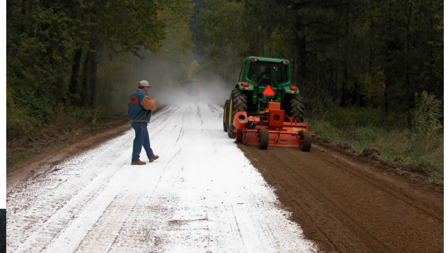
Figure 2.2b—Mixing dry chloride.
