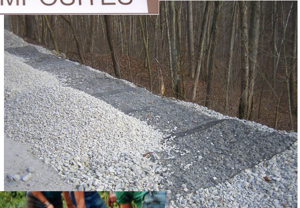
Figure 3.1e— Polymeric Geogrid used on a slip-repair project on a paved road in the developed recreation area, Wayne NF (Cindy Henderson).
