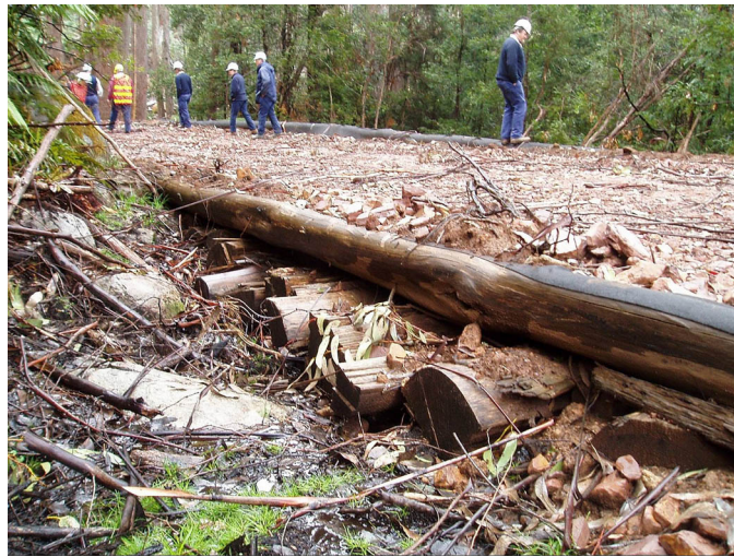
Figure 3.6—Corduroy atop geosynthetic, Australia (Gordon Keller).
