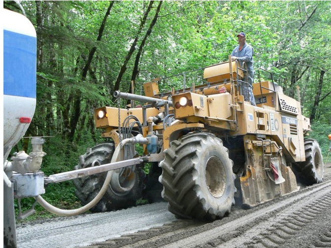
Figure 4.1b— Cement application, region 6 (Dave Katagiri).
