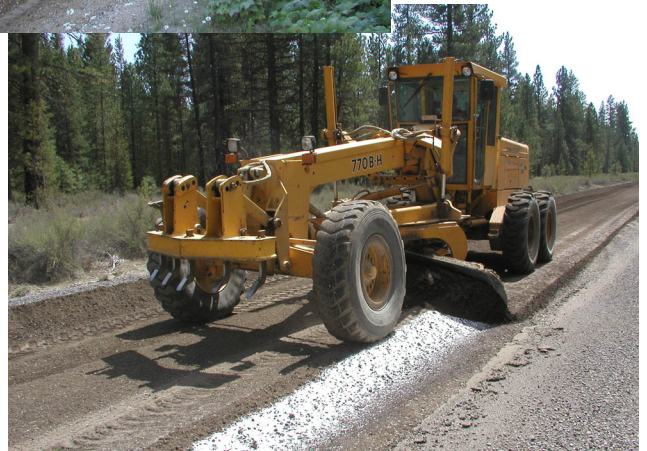
Figure 2.2d—Blade mixing dry chloride.
