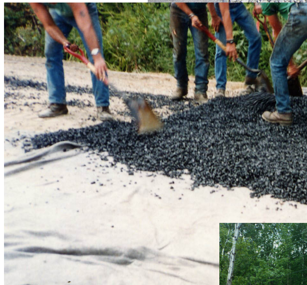
Figure 3.1f— Geosynthetic used immediately beneath asphalt.
