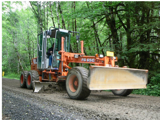
Figure 4.1d— Grading cement-treated base, region 6 (Dave Katagiri).
