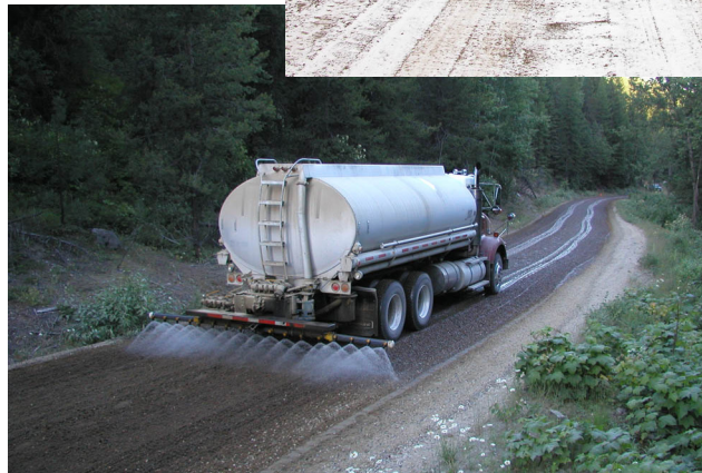
Figure 2.2c—Liquid chloride application.
