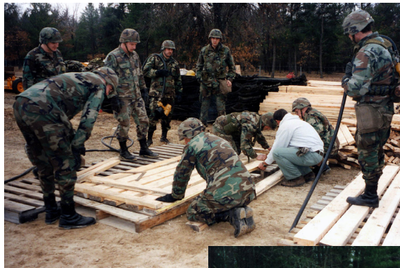
Figure 3.4a— Wood mats being constructed by Forest Service and Wisconsin National Guard (Kestler et al. 1999).
