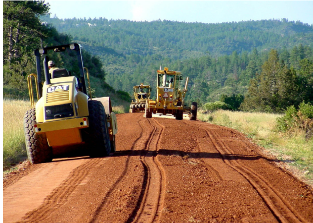
Figure 2.3a— Spreading and compacting.
