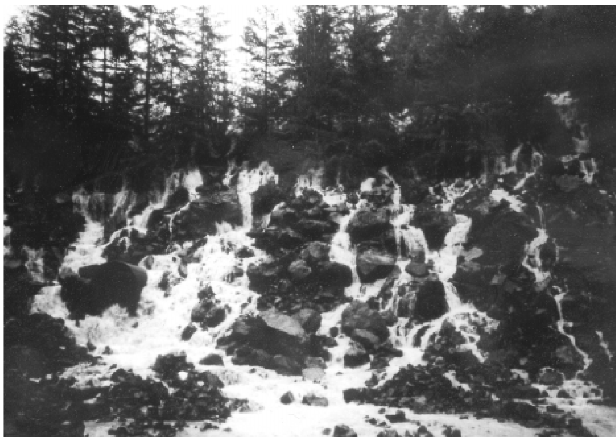
Figure 12—Overtopping of the fill resulting in erosion of the roadway. Understanding the mechanisms that caused failure is useful for upgrading sites to avoid similar consequences in the future.
