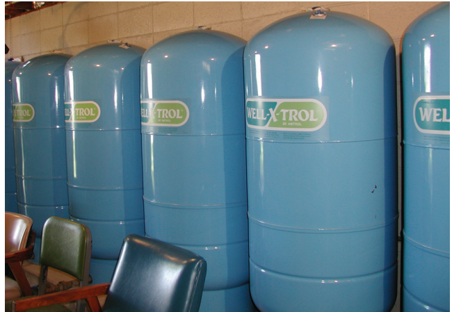
Figure 31—Pressure tanks.
