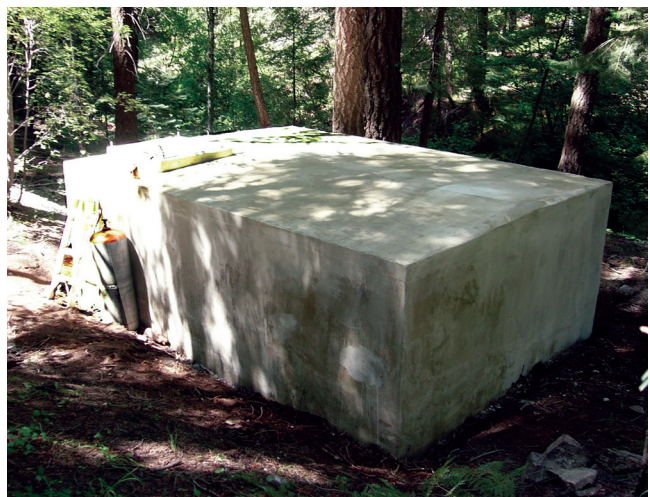
Figure 33—Concrete water tank.
