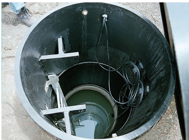
Figure 37—This buried tank access needs a confined space warning and a lock for security.
