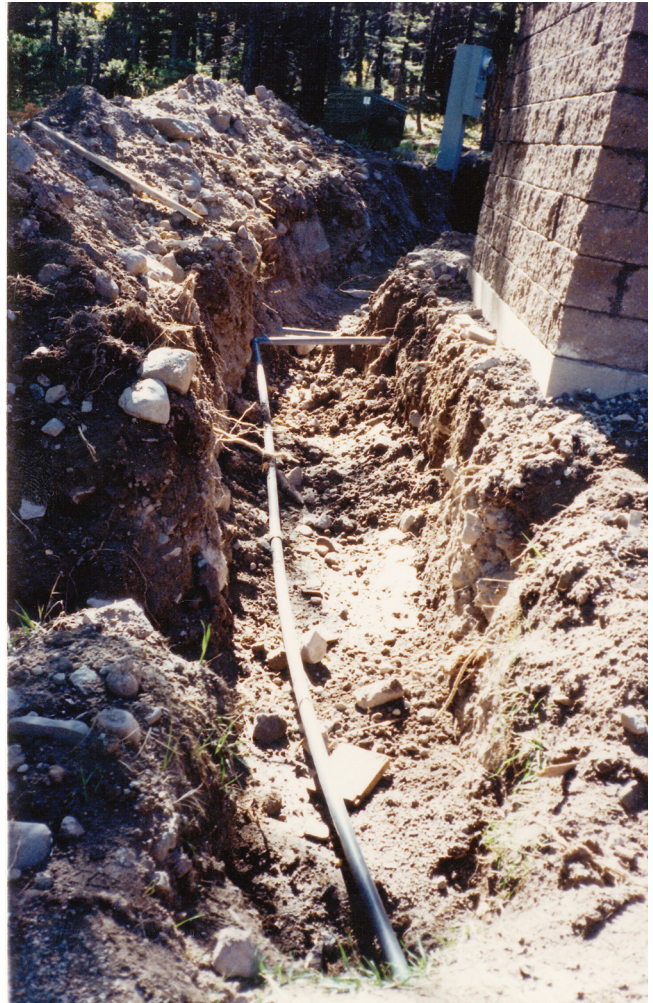
Figure 39—Distribution system pipe placed in a trench.
