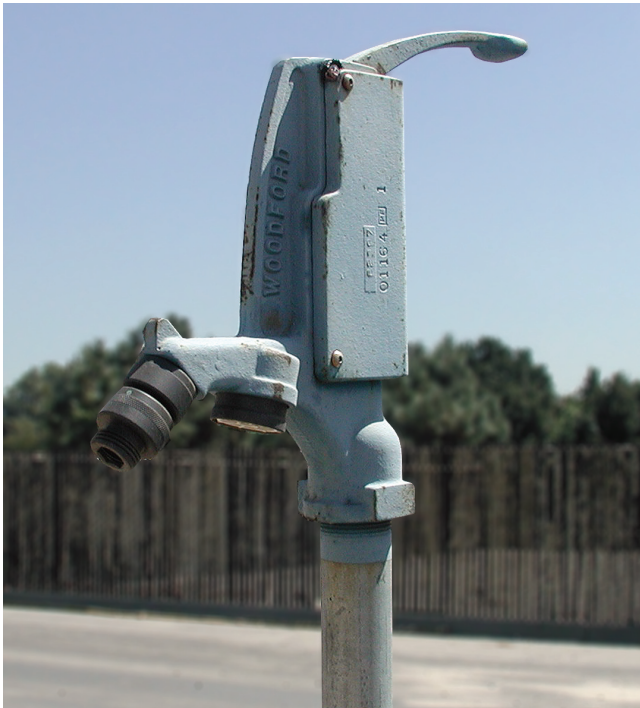
Figure 44—Freezeproof hydrant.
