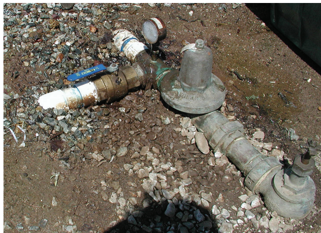
Figure 42—Leaking valve.
