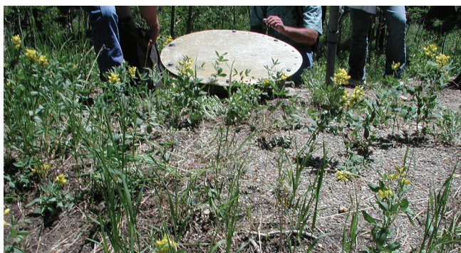
Figure 35—Tank lids must be locked. Replace two opposing bolts with padlocks for security.
