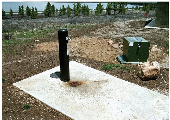
Figure 46—Faucet with concrete pad and drain.
