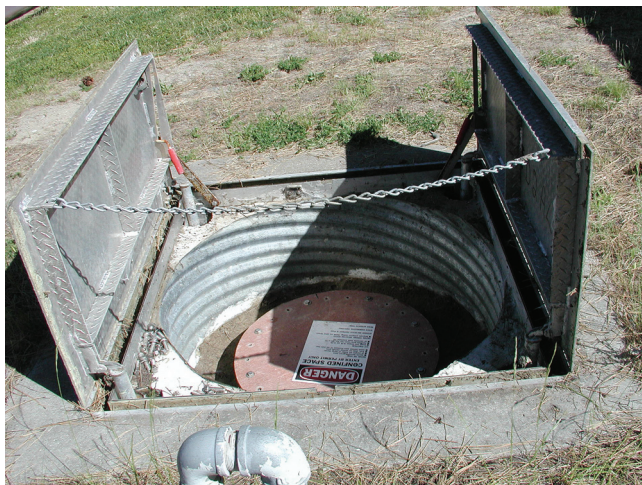
Figure 36—Access to a buried water tank. The outer hatch doors are hinged with a lock. A confined space warning is clearly posted.
