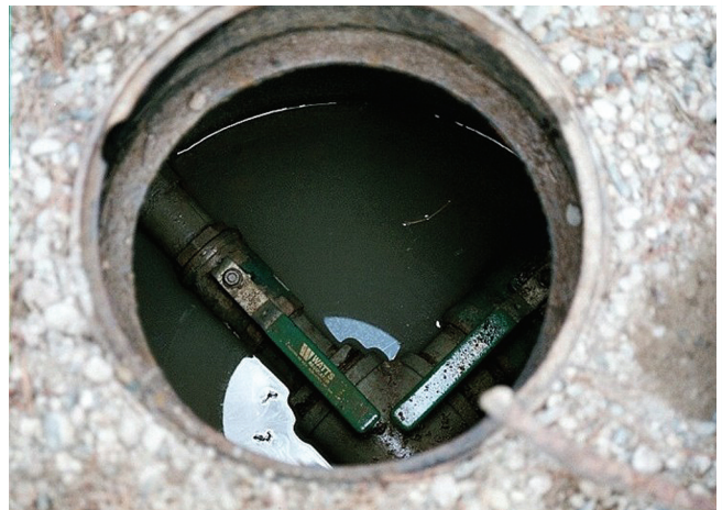
Figure 40—Valve box.
