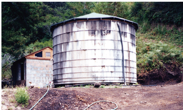
Figure 34—Wooden water storage tank.
