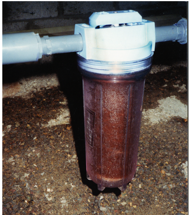
Figure 74—Small cartridge filter.
