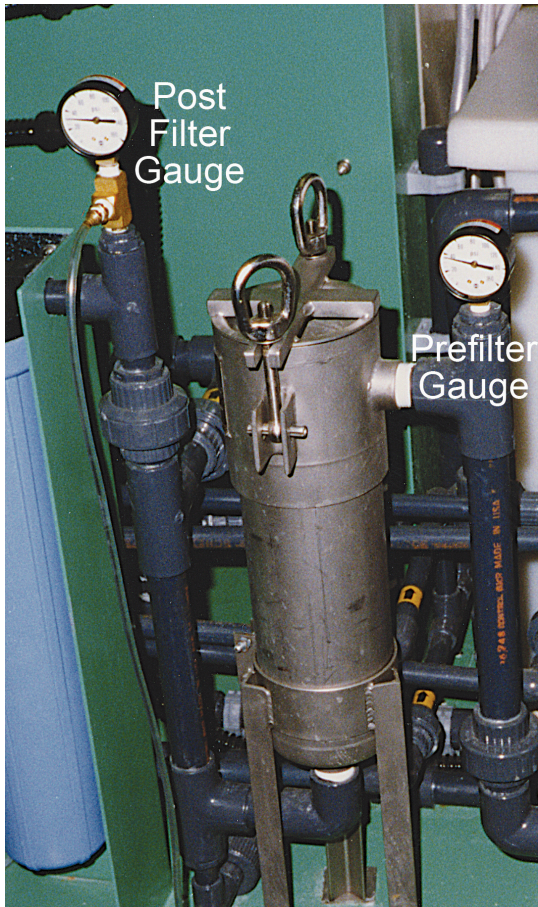
Figure 79—Pressure gauges installed before and after a bag filter.
