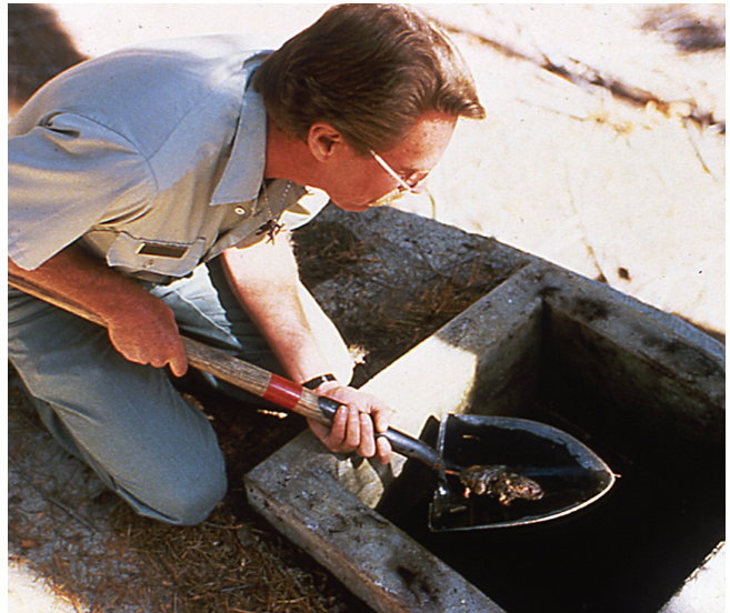
Figure 86—Tank contaminated by a dead rodent.
