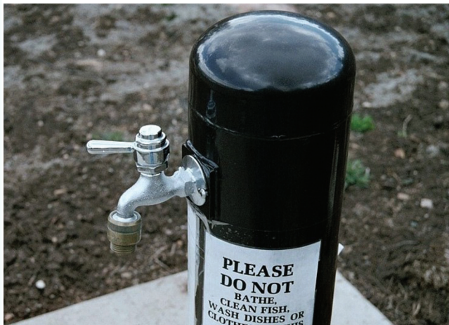
Figure 84—Atmospheric vacuum breaker.
