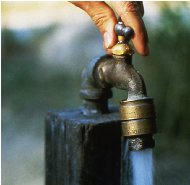
Figure 53—Open each hydrant until chlorine is detected.
