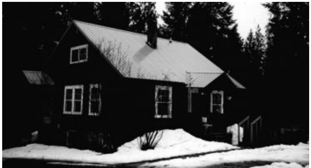
Figure 8. Residence Number 2 at the West Fork Ranger Station.
