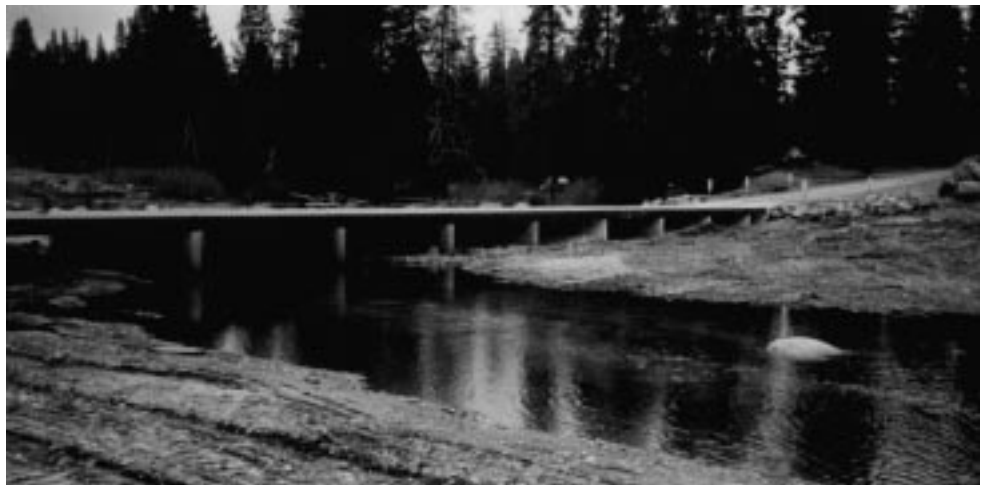
Figure 2. Jones Wreckum Crossing looking downstream from the east.
