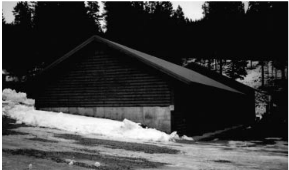
Figure 2. The West Fork Ranger Station's garage.
