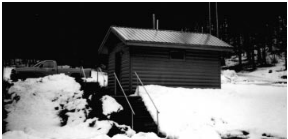
Figure 5. The West Fork Ranger Station's laundry.
