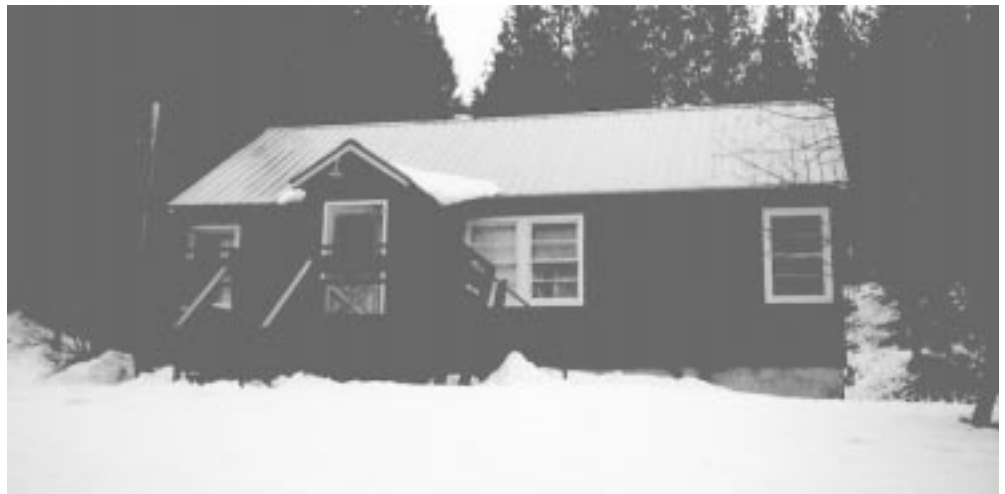
Figure 7. Residence Number 1 at the West Fork Ranger Station.
