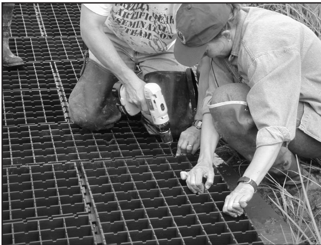
Figure B7—Joining the sections using a screw gun. Note the underlying plywood.
