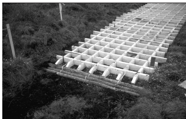
Figure 17—Wood matrix after installation in the Wrangell-St. Elias National Park and Preserve in Alaska. The wood matrix provided a suitable surface for OHVs, but had several characteristics that limited its suitability for future field applications.
