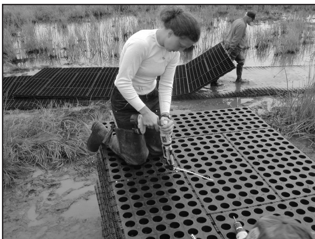
Figure B4—Assembling the subsections with the Quik Drive drill system. Using this tool and a standard 18-volt cordless drill, two people can assemble 32 six-panel subsections in 1½ hours. In the background, a worker drags a three-section assembly along an installed trail segment.
