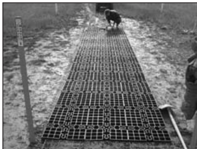
Figure 24—Test installation of SolGrid at the Palmer Hay Flats State Game Refuge in Alaska. Note the U-shaped flex joints between sub-panel sections. The SolGrid was tested without Polynet PN-3000 to test the characteristics of the product when installed on a soft, silty substrate.
