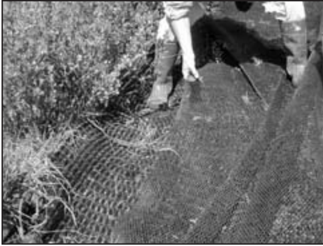
Figure 14—Polynet over Pyramat was used in this National Park Service installation to test the addition of a synthetic turf reinforcement mat. The Polynet, with its more durable wear surface, was installed over the less durable Pyramat.
