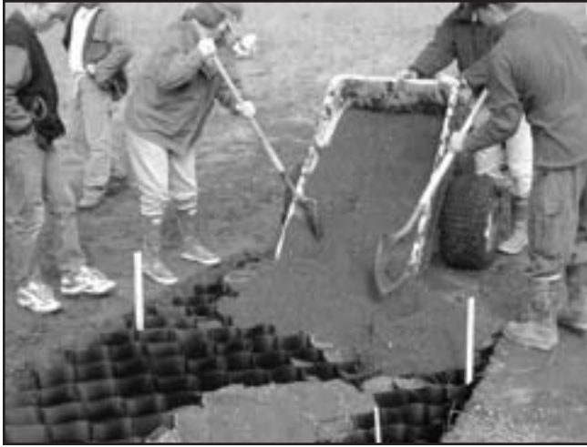
Figure 13—A cellular confinement system being installed on an experimental trail in southcentral Alaska. Four-inch-deep cells were formed by expanding the cellular product accordion style, then backfilling and compacting with a suitable fill material—in this case, sandy gravel. The sides of the installation were confined by a 6-inch-deep trench.
