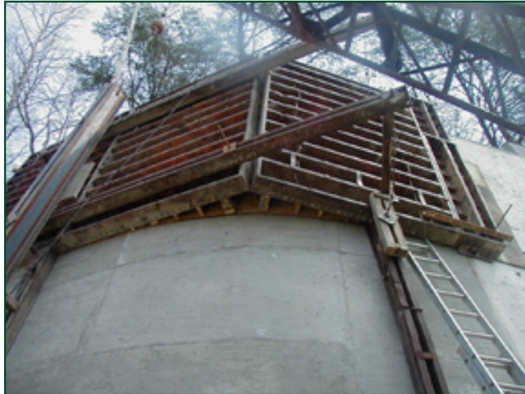
Figure 5—Forming a curved section of spillway wall.
