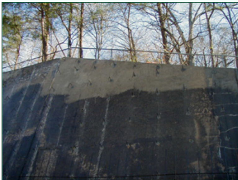
Figure 4—Grouted anchor bars installed in old spillway walls.
