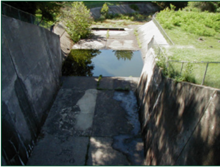
Figure 1 — Stilling basin of spillway before new concrete is installed.
