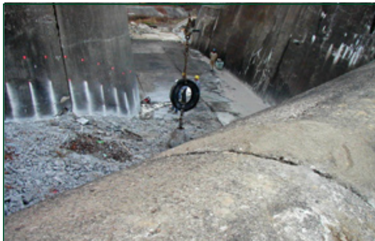
Figure 3—Wrecking ball on crane used to break up the spillway floor.
