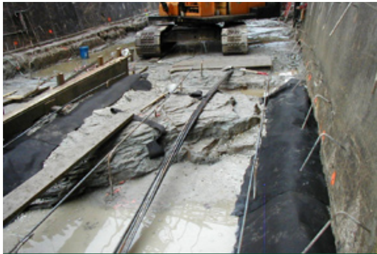
Figure 2—Exposed bedrock under the spillway floor with grouted anchor bars installed.
