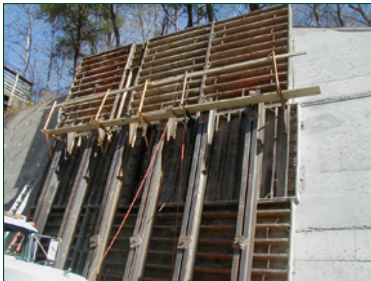
Figure 6—Steel forms used to form spillway walls.
