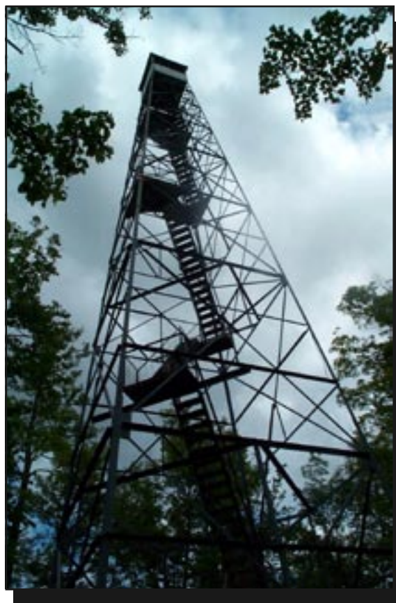
Figure 7—The Horn Lookout Tower in the St. Francis National Forest is a standard steel lookout tower built in the early 20th century.
