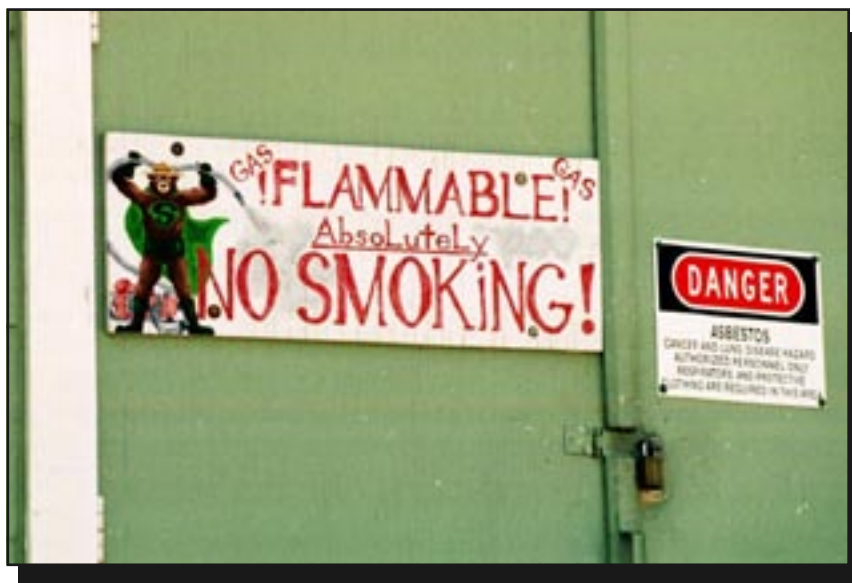
Figure 4—This flammable materials sign, while amusing, doesn’t meet the required standards.
