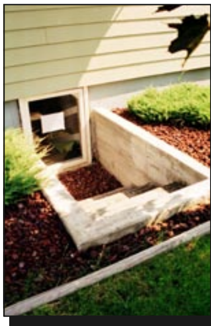
Figure 6—This basement egress window at the Bitterroot National Forest's Darby Ranger Station meets code requirements.
