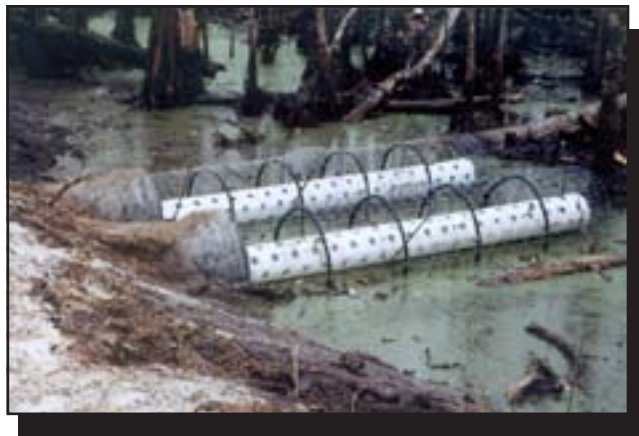
Figure 14—The Clemson Beaver Pond Leveler uses a perforated PVC pipe for water intake and a reducer to limit waterflow through the output pipe.
