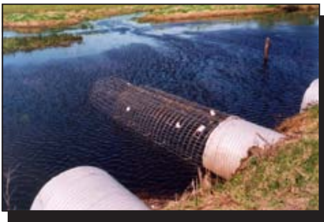
Figure 10—The Beaver Stop wire mesh culvert extension.—Courtesy of FSI Culvert, Inc.
