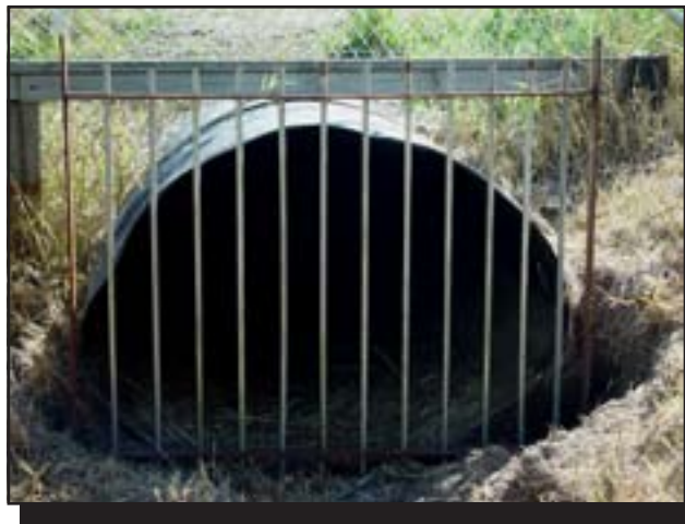
Figure 5—This beaver guard is constructed by inserting steel rods through a frame mounted on the front of a culvert.
