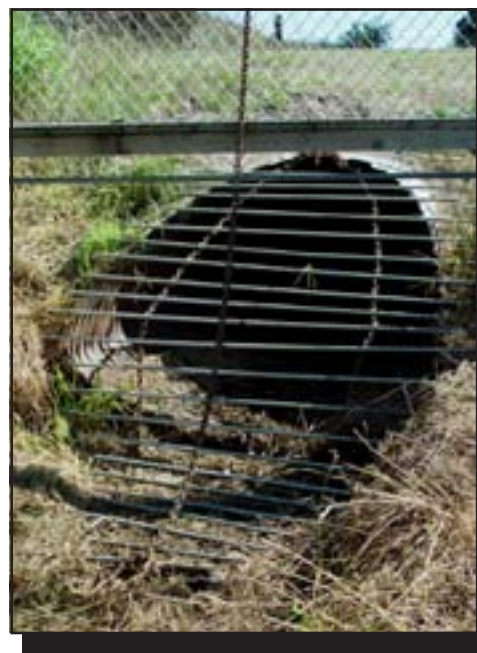
Figure 6—This beaver guard has chains that allow the guard and any debris that collects on it to be pulled up over the culvert.
