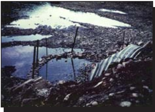
Figure 8—A rounded fence can help keep beavers from damming a culvert.
