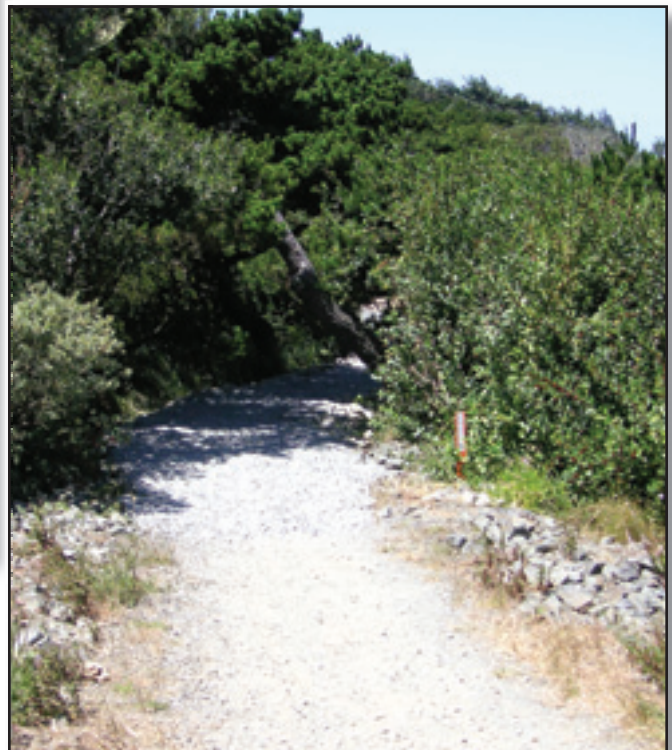
Figure 22 —A finished rock and geotextile underdrain.
