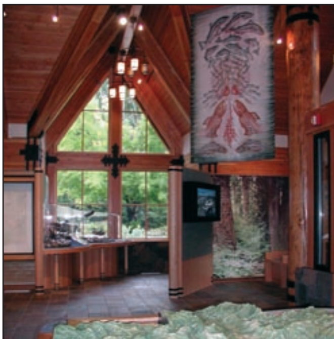
Figure 8—The durable wood walls and slate floors of the visitor information center and entry to the McKenzie River Ranger Station although initially expensive, will stand up to the demands of high visitor use far longer than less durable materials (Willamette National Forest, Pacific Northwest Region).
