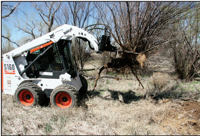
Figure 4—The Bobcat S160 skid steer loader.
