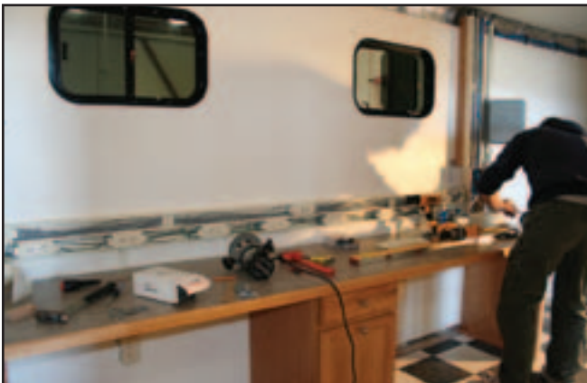
Figure 7—MTDC employees installed custom cabinets and other components inside the MIMIT trailers. Electricians installed the power and network wiring. The trailers were delivered to NIFC in May 2009.
