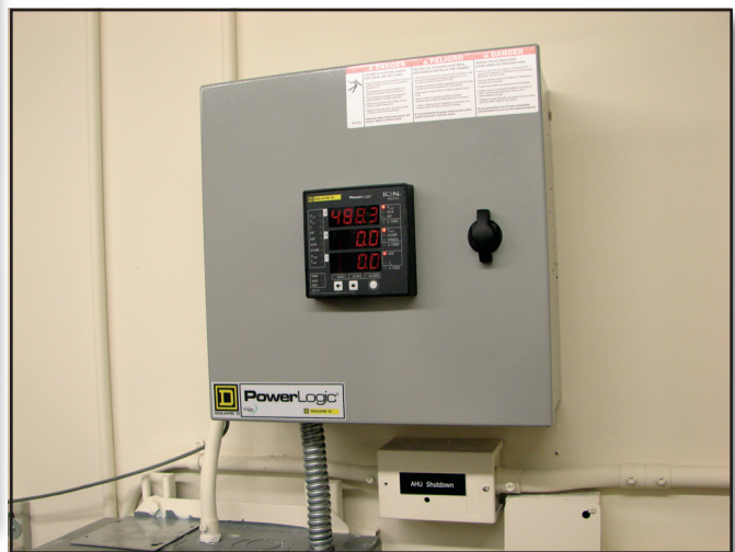
Figure 5—A typical low-end submeter that sends data to a high-end meter that stores the data.
