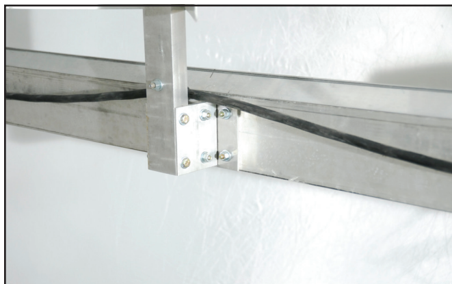
Figure 10f—The electrical wire is routed along the side of the rail.
