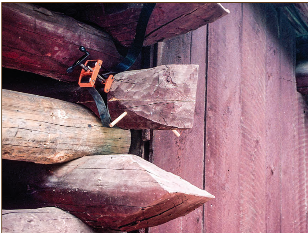
Figure 174—Preservation crewmembers removed the bottom of a crown end log on the barn at the Moose Creek Wilderness Station (Nez Perce National Forest, Northern Region) to free the log below it for replacement. The new log (lighter color) is in place. The piece that the crew removed is glued and doweled back into position and is held in place by a band clamp while the epoxy adhesive cures. Next, the crew will trim the dowels and stain the replacement log and dowel ends to match the existing logs, providing a nearly invisible repair.
