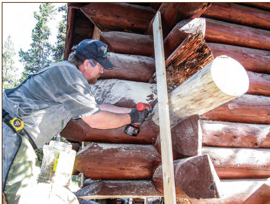
Figure 184—Kirby Matthew, now retired from the Forest Service Northern Region Historic Preservation Team, drives one of two temporary screws. He's using the screws, a tie board, and epoxy adhesive to hold the replacement crown end in place while he drills holes for the permanent dowel connection.
