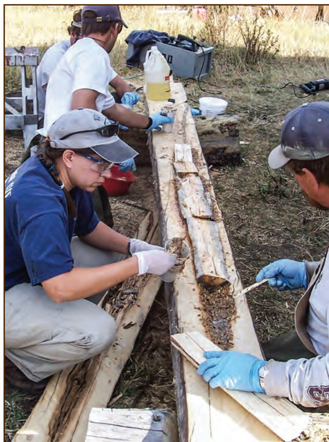
Figure 159—Preservation crewmembers chiseled out the rotted interior of this heavily coped log at Badger Cabin (Lewis and Clark National Forest, Northern Region). The author (left front) and crew replaced the removed material with epoxy, sawdust, and wood slabs. The rot was more extensive in the center of the log than at the ends. The outside of the entire log was sound. The crew split the log in half so that they could repair the interior, then rejoined the log using techniques in the Structural Wood Splicing section of this guide.
