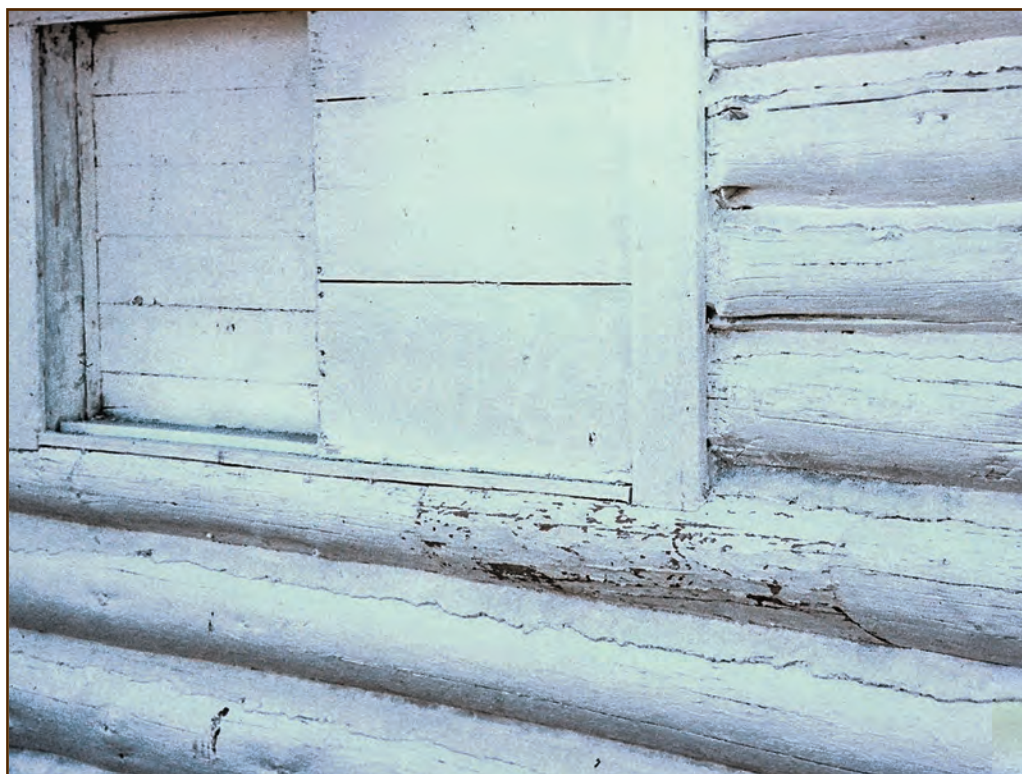
Figure 173—The preservation carpenter has repaired the chinking and daubing and applied whitewash to the patch, which is just barely noticeable. The whitewash didn't penetrate the new splice as well as the original logs. By the time the cabin needs another application of whitewash, the splice will have weathered and will absorb the whitewash more uniformly.
