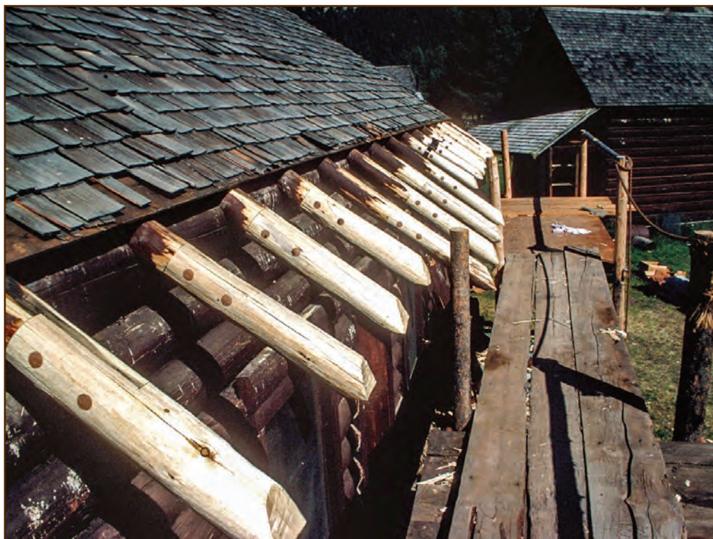
Figure 191—Preservation crewmembers replaced all the rafter tails on this building. The crew trimmed the dowels flush with the rafter tails, but the dowels still are clearly visible as darker spots. Next, the crew will stain the rafter tails using the same product as the original rafter tails. Finally, they will install new sheathing and roofing.
