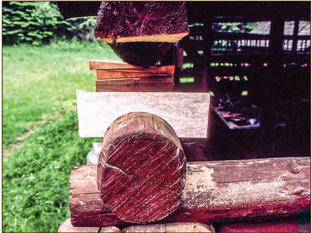
Figure 157—You can use a cardboard pattern to scribe the outline for mid-wall saddle notches.
