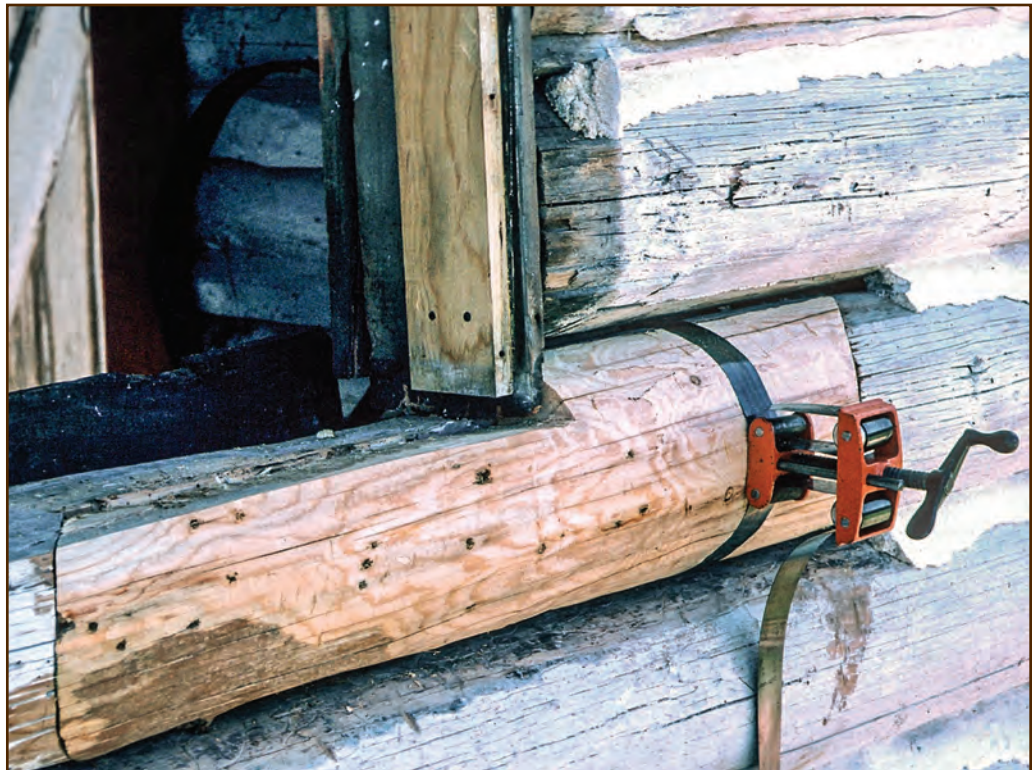
Figure 171—The preservation carpenter removed the original windowsill and cut the top of the splice down for the windowsill. He applied epoxy adhesive behind the patch and secured the splice to the original wall with a band clamp. The splice fit perfectly into the notch. Next, he drilled the dowel holes.
