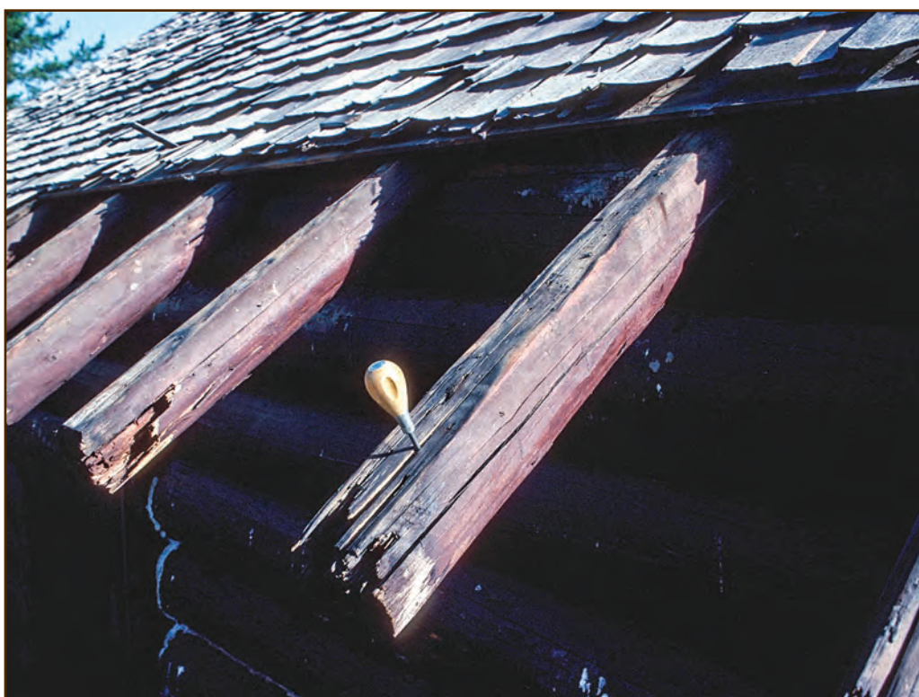
Figure 186—Preservation crewmembers removed the sheathing and roofing from these rotted rafter tails. The penetration of the awl into one of the rafter tails shows the depth of the rot. The crew will have to remove about a foot from the ends of these rafters.
