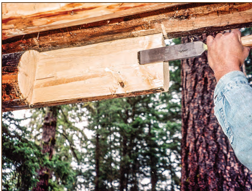
Figure 188—A preservation crewmember used a saw to cut the shape for a half lap joint on this purlin end, and a chisel to smooth the face flat.
