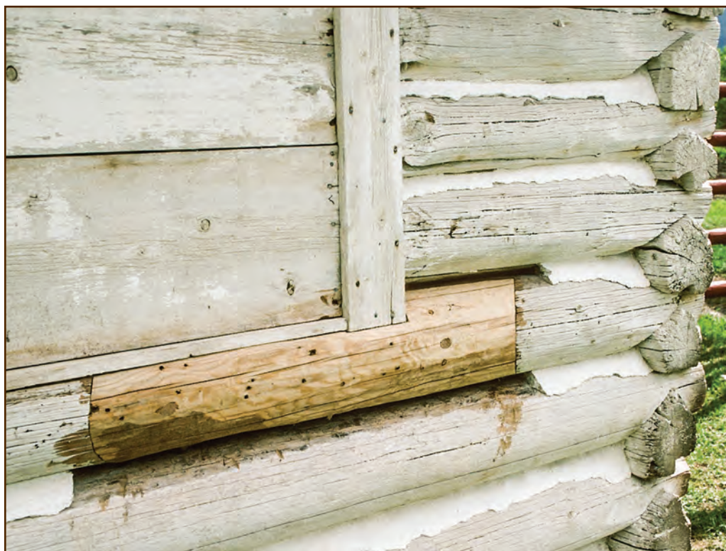
Figure 172—The ends of the angled dowels are darker ovals that are visible toward the ends of the splice. The epoxy has cured and the preservation carpenter has removed the band clamp.
