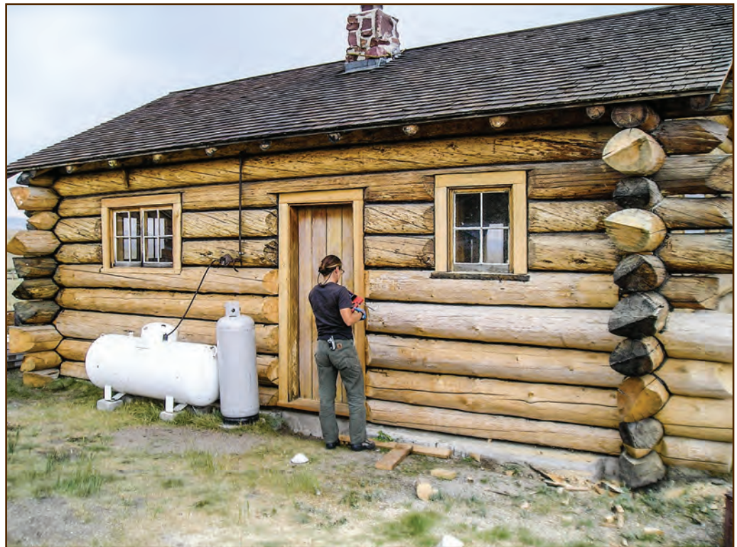
Figure 194—This worker is using a caulking gun to apply tar daubing between the logs of the Horse Prairie Cabin (Beaverhead-Deerlodge National Forest, Northern Region).
