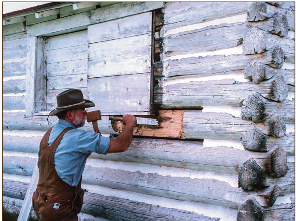
Figure 167—Preservation carpenter Bernie Weisgerber, now retired from the Forest Service Northern Region Historic Preservation Team, used a mallet and chisel to remove the deteriorated wood, which was more extensive than it appeared at the surface. Notice that he removed the chinking and daubing adjacent to the deteriorated area so that he could more easily access the damaged area.
