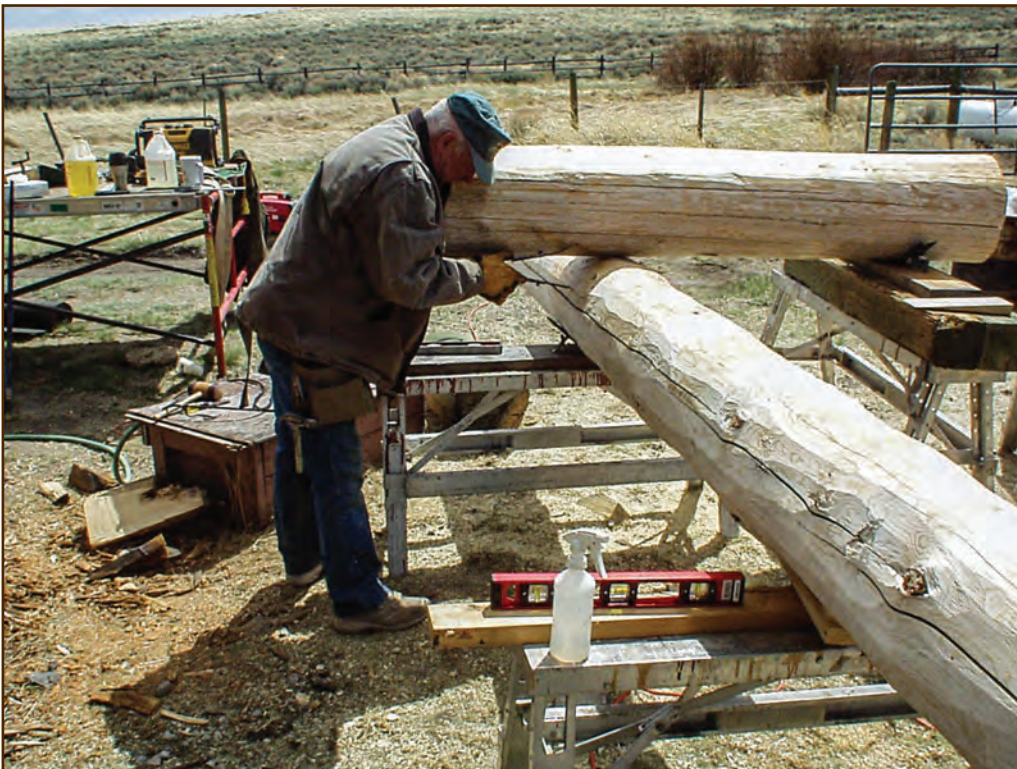
Figure 158—This preservation crewmember is using a log scribe and a dummy log to make a saddle notch for the Horse Prairie Cabin in the Beaverhead-Deerlodge National Forest, Northern Region.
