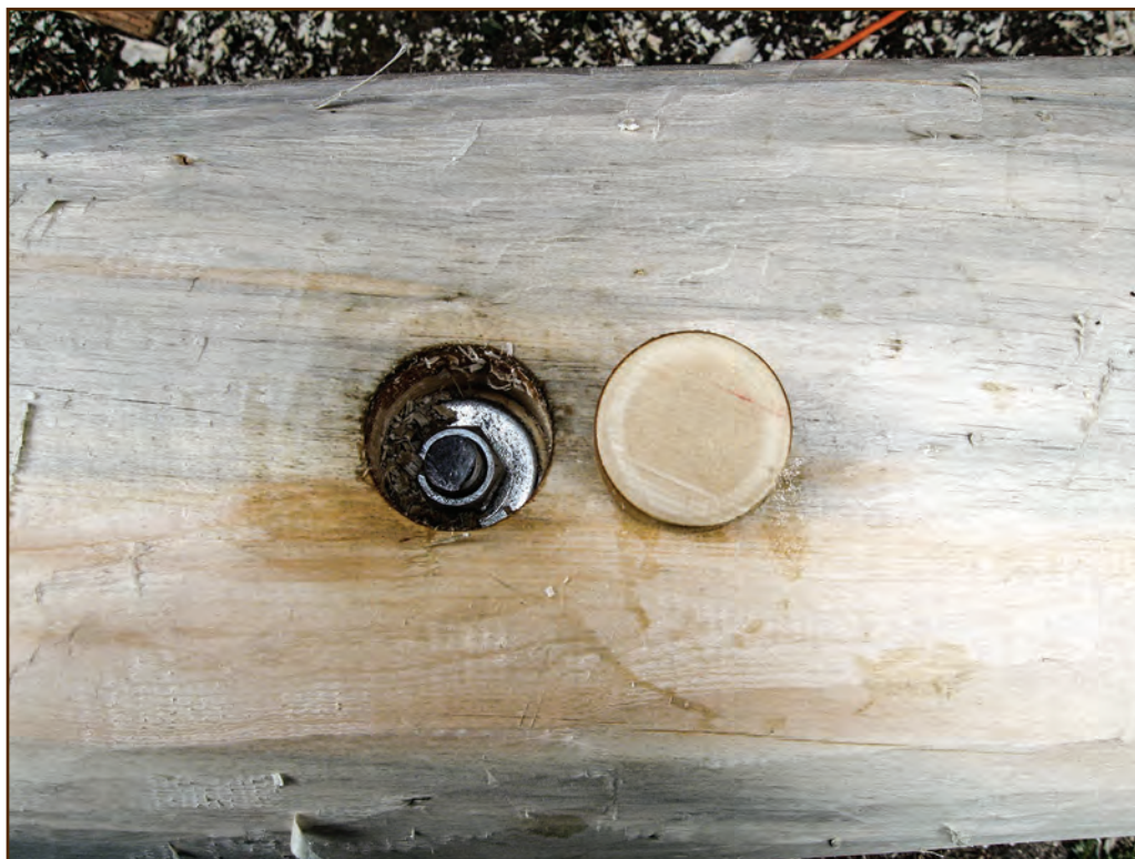
Figure 180—This closeup photo of the outside of a spliced log shows the recessed bolt, nut, and washer of a split-ring connector. The plug that the preservation crew will glue in place to cover the recessed bolt and nut sits on the log beside the recess.
