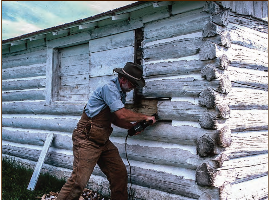
Figure 168—The preservation carpenter used a reciprocating saw to cut a clean edge at an angle on the end of the cut out area.
