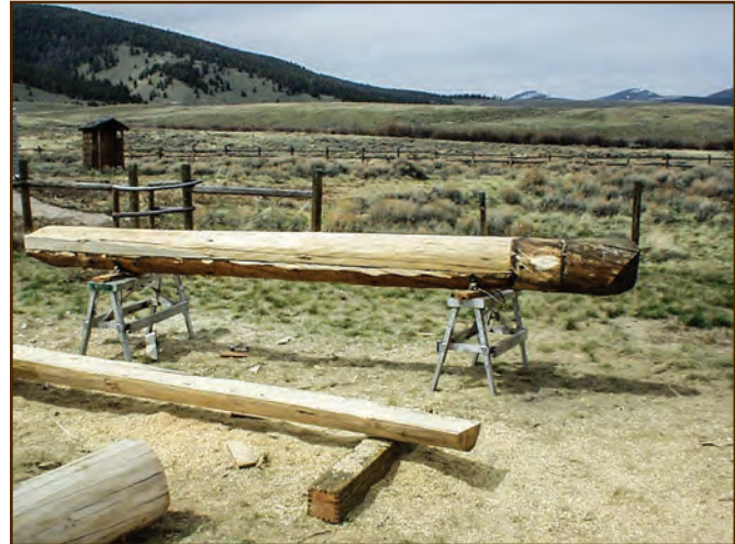
Figure 177—This photo shows a half-log splice in progress. The crew has not yet completely shaped the pale new wood to match the wood it will replace. This splice doesn't include the end of the existing log because the end was sound, and the crew didn't need to repair it. Using a half-log splice allowed the crew to keep the historic interior finish intact. It is always best to retain as much historic material as possible.
