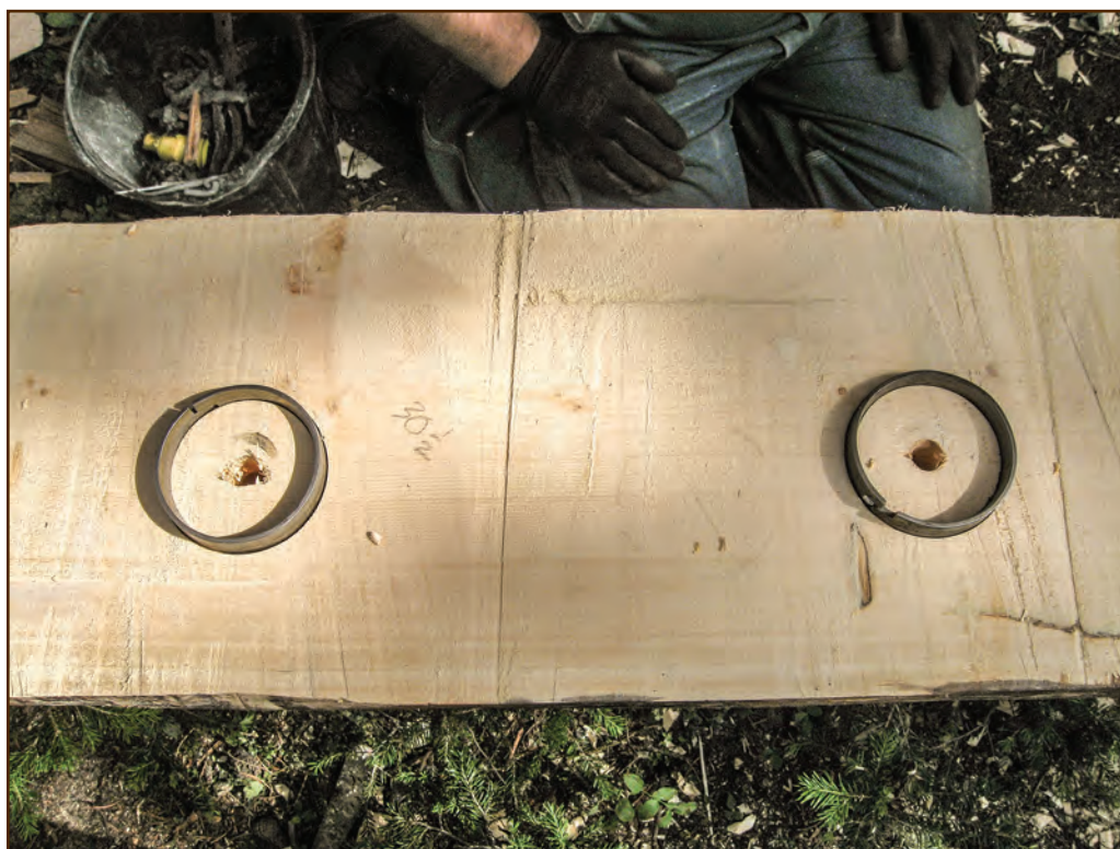
Figure 179—Preservation crewmembers recessed split-ring connectors halfway into this splice. They also will recess the connectors halfway into the old log. Next, they will put the splice and log together, thread the bolt through the matching center holes in the splice and old log, and secure the connection with nuts and washers.
