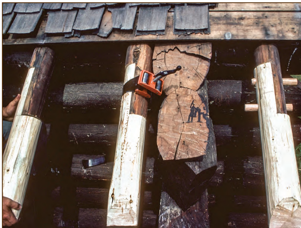
Figure 190—This photo shows three stages of rafter tail replacement using a lap joint. On the left, a preservation crewmember checks the fit of the replacement rafter tail. In the middle, the crewmember applied epoxy adhesive to the cut faces of the existing log and clamped the replacement rafter tail in place. On the right, he inserted the glued dowels into the drilled holes.
