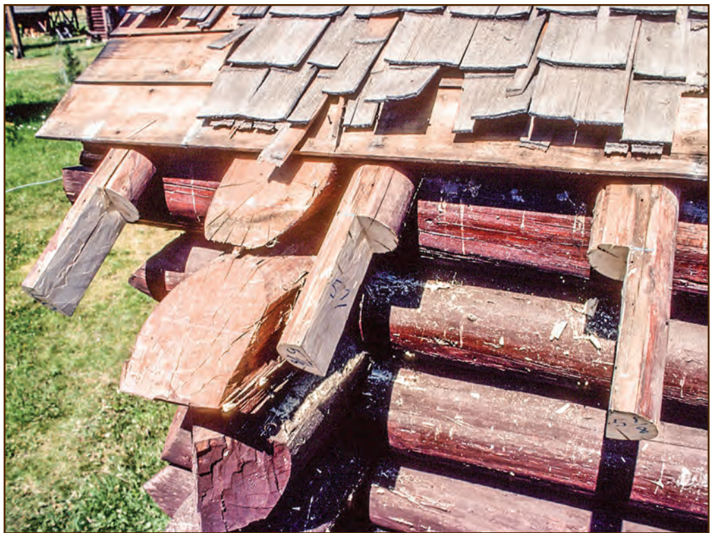
Figure 189—Preservation crewmembers cut these rafter tails to the same pattern to make shaping and attaching the replacement rafter tails easier. They oriented the joints with a vertical splice cut to maximize the strength of the joint and to allow any water that might enter the joint to drain.
