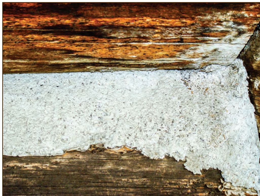
Figure 195—The daubing on this Wyoming Game and Fish cabin in Sunlight Basin appears to contain tiny fossilized seashell fragments from the local limestone. To duplicate the appearance of this daubing, you'll need to locate the source and use the same material when you mix daubing for repairs.
