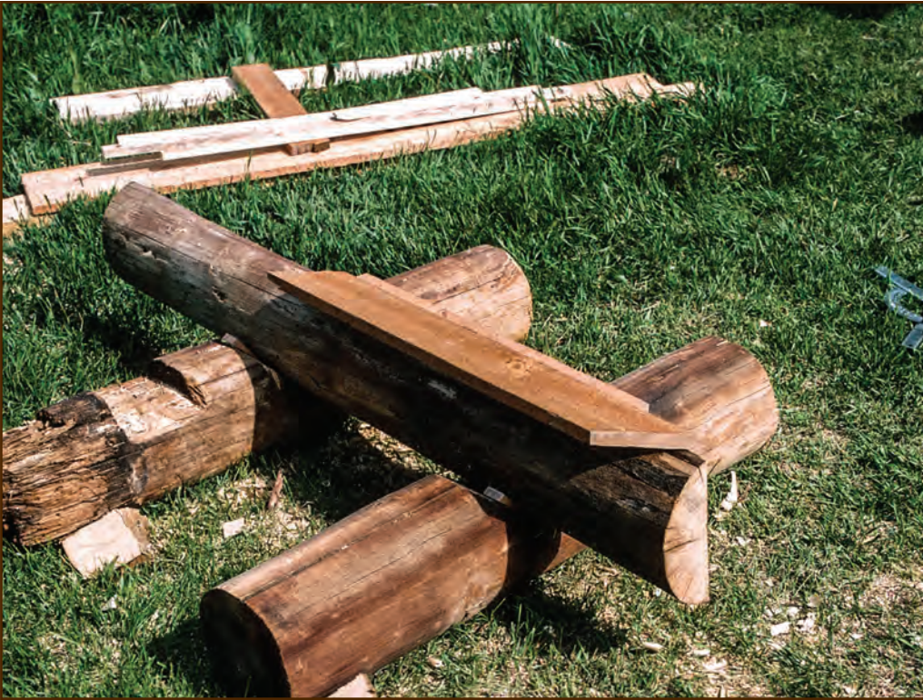
Figure 170—The preservation carpenter cut a board to match the length and angles of the cut out area as a pattern for cutting the splice.
