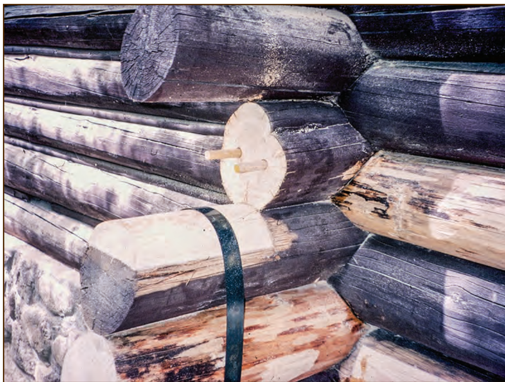
Figure 181—This cabin with battered crown ends required several crown end repairs. Preservation crewmembers have completed two full crown end replacements and a splice and have begun a partial crown end replacement. They have inserted the dowels into the original log and will attach the replacement end next.
