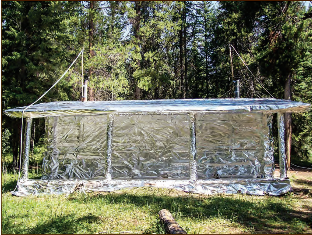
Figure 218—Preservation crewmembers completely wrapped the Kenck Cabin (Lewis and Clark National Forest, Northern Region) with fire resistant material as the 2007 Ahorn forest fire approached. The poles attached to the flues support sprinklers, and the white “ribbons” trailing from the top of the poles are fire hose. The cabin survived unscathed.
