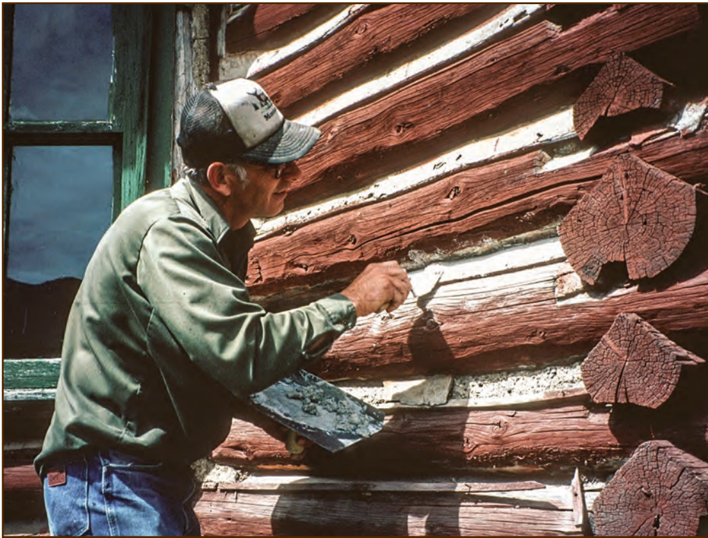
Figure 200—This preservation crewmember is using a small trowel to apply daubing to a cabin, carefully matching the profile of the new daubing to that of the original daubing. His hawk is nearly empty of daubing material.
