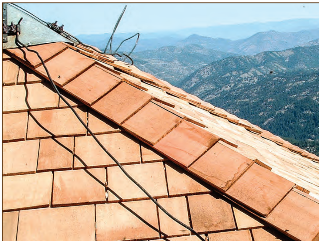
Figure 227—The shingle hip cap shown in this photo is a common style used on square, shingle-roofed lookouts in the Northern Region.
