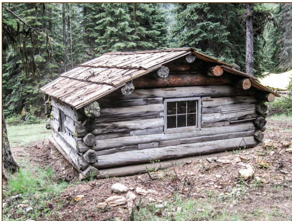
Figure 222—This 1920 storage building at the Greenwood station in the Lolo National Forest of the Northern Region needs extraordinarily long shakes to span the spacing between purlins.
