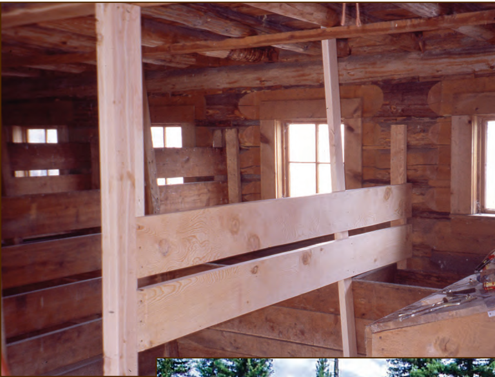
Figure 207—The builders used tie beams (that also served as ceiling joists) on the two-story Steel Creek Barn (Beaverhead-Deerlodge National Forest, Northern Region) to ensure that the walls wouldn't spread apart over time because of pressure from the rafters.
