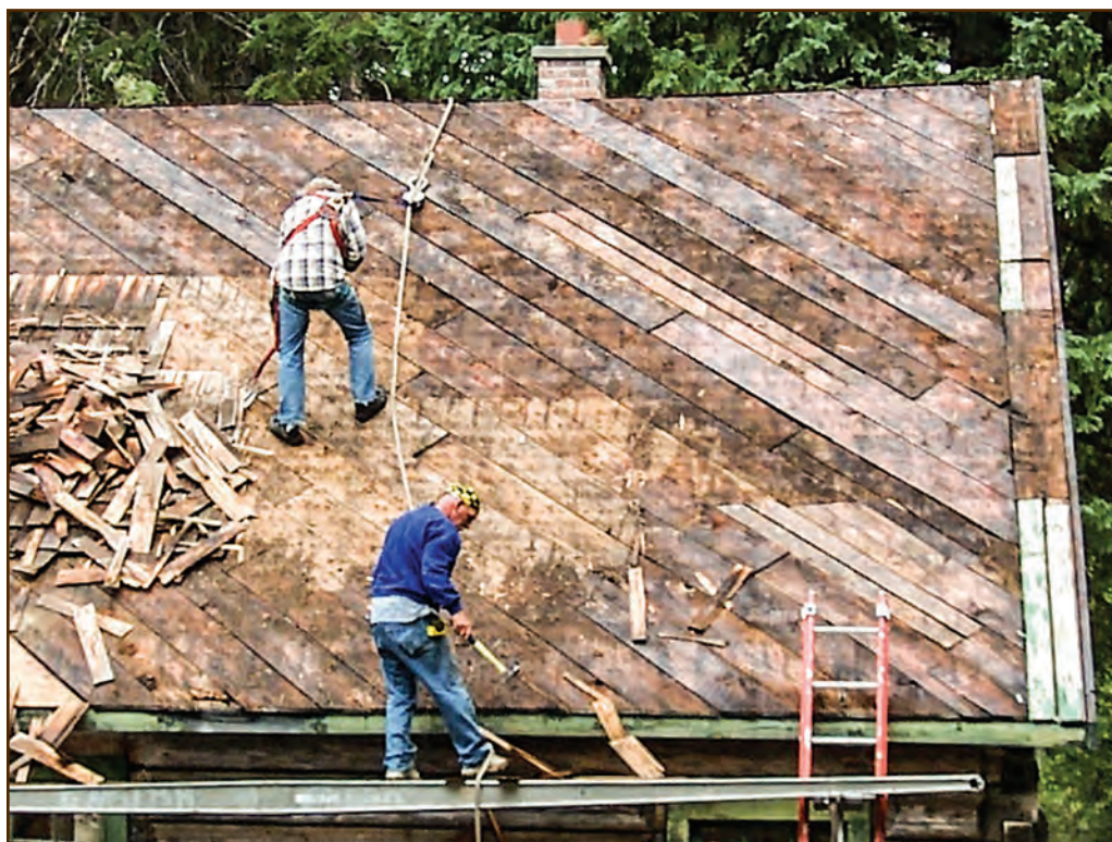
Figure 212—The sheathing on the one-and-a-half-story Adams Camp Ranger's House, built in 1933, consists mainly of diagonal 1-inch-thick boards with vertical boards at the gable overhangs. The varying widths and colors of the sheathing boards provide evidence of various repairs made over the years. Adams Camp is located in the Salmon River Ranger District of the Nez Perce National Forest in the Northern Region.
