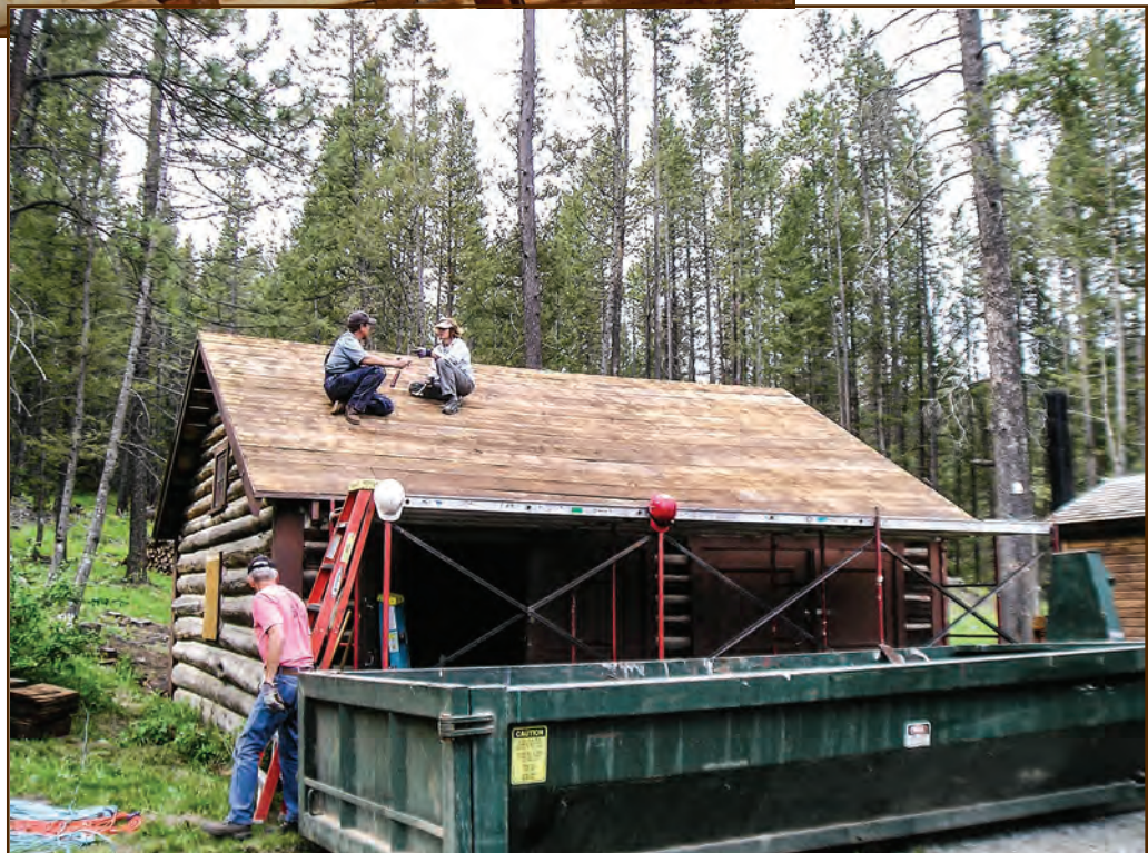
Figure 210—The roof sheathing on the Moose Creek Station garage (Helena National Forest, Northern Region), built in 1930, is 1-inch-thick boards applied horizontally over the rafters.
