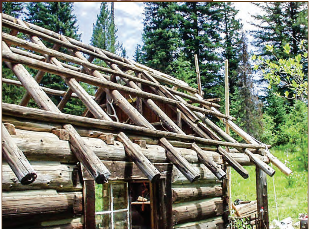
Figure 208—The Liz Creek Cabin (Clearwater National Forest, Northern Region) has a rafter and purlin roof structure. Because of decay, preservation crewmembers removed one of the purlins and the roofing, revealing the framing. They replaced these components before installing the new roofing.
