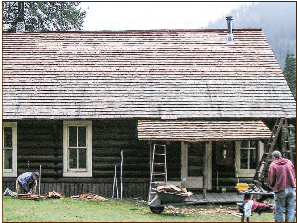
Figure 224—The cock's comb ridge cap is clearly visible on the skyline of the newly reroofed Office/Cookhouse building at the Moose Creek Wilderness Station (Nez Perce National Forest, Northern Region).
