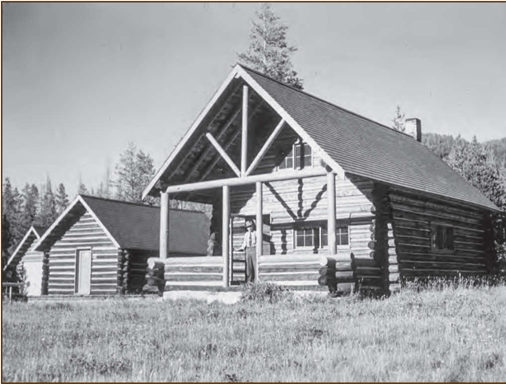
Figure 204—A simple king post truss constructed of logs supports the porch of the cabin at the Stolle Meadow Guard Station (Boise National Forest, Intermountain Region). The cabin has a cedar shingle roof. This photo was taken in 1939, not long after the builders constructed the cabin. The cabin still is in use today.
