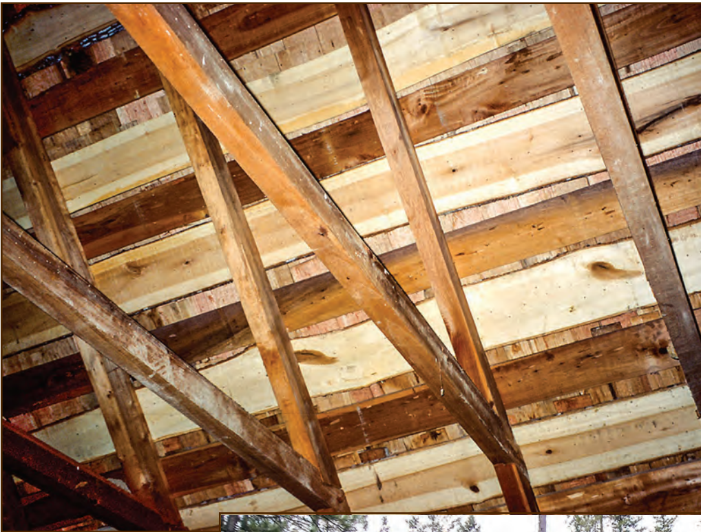
Figure 209—The spaces between the sheathing boards are clearly visible in this photo of the underside of a cabin roof. Roofers added new sheathing boards (lighter color) between the darker color original sheathing boards before putting new shingles on the roof. The shingles are visible in the gaps between sheathing boards. Spaced sheathing often is referred to as “skip sheathing” or “shingle lath.”
