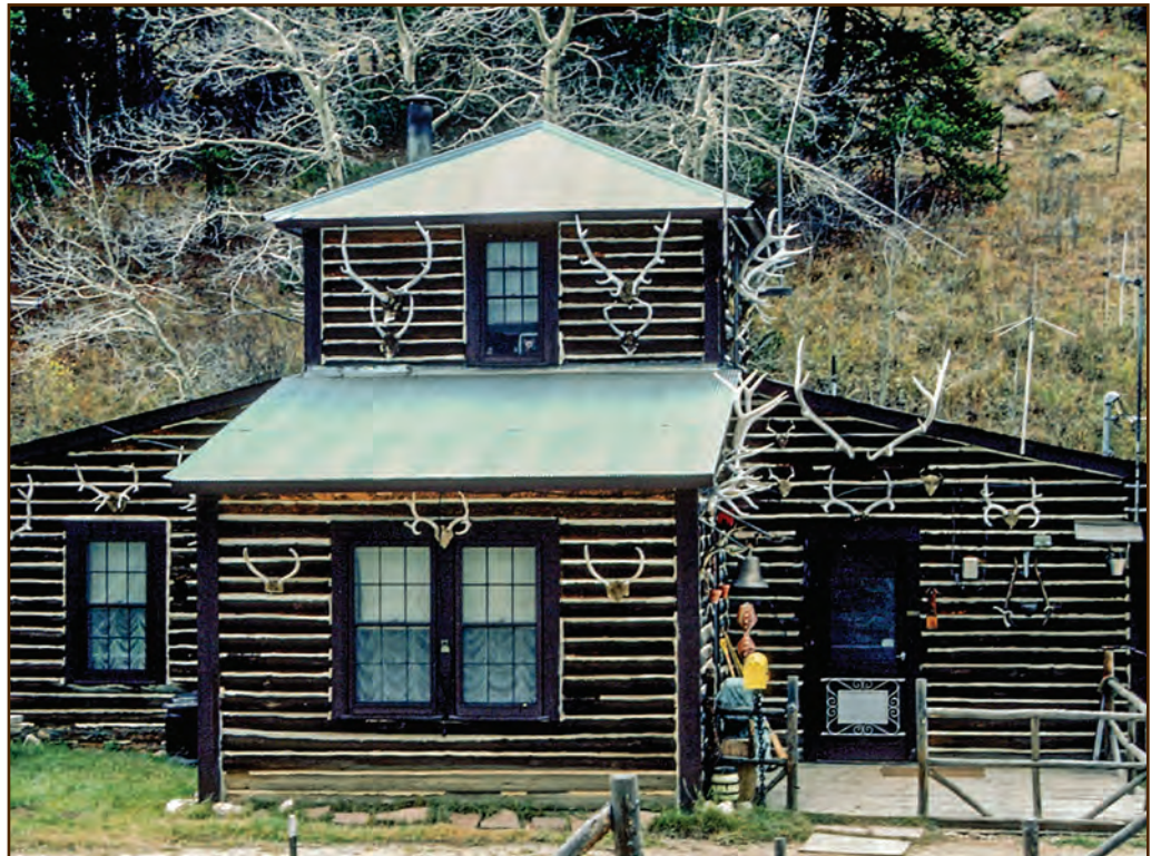
Figure 230—This fancy log house has corrugated galvanized steel panel roofing. Roofers used matching galvanized steel ridge covers on the pyramidal second floor roof.
