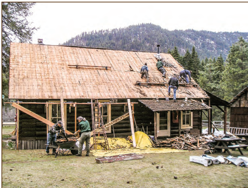
Figure 211—The roof sheathing on the Office/Cookhouse building at the Moose Creek Wilderness Station (Nez Perce National Forest, Northern Region), constructed in 1921, is 1-inch-thick by 12-inch-wide boards applied vertically over the purlins. This photo shows the south side of the building.
