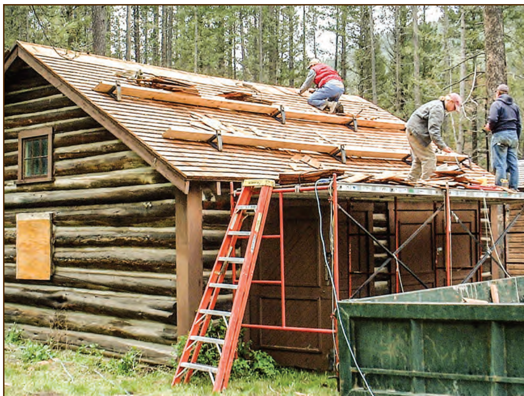
Figure 202—These roofers placed planks on roof jacks, providing a secure surface for their feet during the reroofing of the Moose Creek garage (Helena National Forest, Northern Region).
