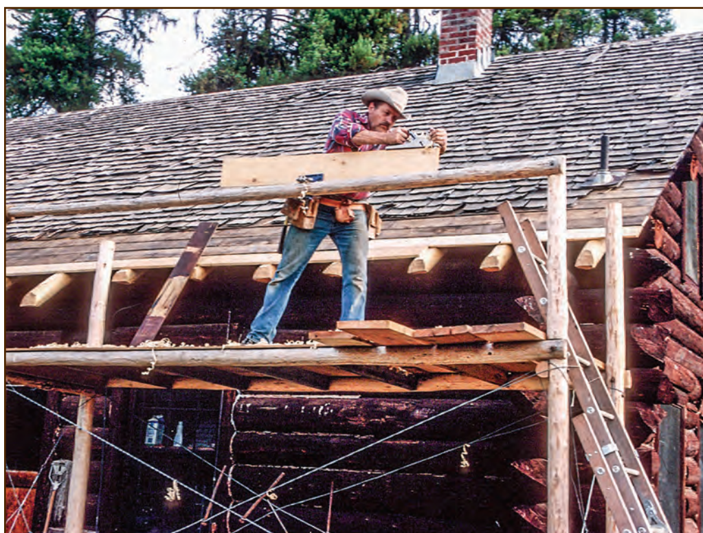
Figure 236—This old photo shows a preservation crewmember planing a replacement sheathing board so that he can fit it properly on the log Ranger Cabin at Big Prairie Work Center (Flathead National Forest, Northern Region). All the rafter tails and the sheathing attached to the tails on this side of the cabin, built in 1933, were rotten; the preservation crew had to replace them.
