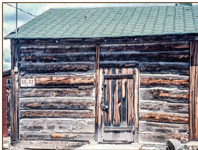
Figure 229—This cabin has an interlocking asphalt shingle roof. Builders have used this interlocking pattern since the late 1920s and still commonly install it on new buildings, particularly in high wind rural areas, because of its wind resistance. An interesting detail on this roof is the bent-over shingles at the roof eaves that function as a sort of inexpensive, integral drip edge.
