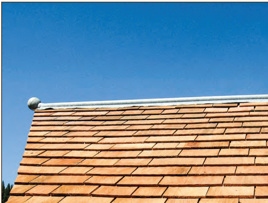
Figure 226—Builders commonly used metal ridge cap on early 20th-century buildings, including log cabins. This photo shows the original metal ridge cap, which preservation crewmembers carefully removed and reinstalled after they replaced shingles on this building at the Ninemile Ranger Station (Lolo National Forest, Northern Region). Most of these premanufactured metal ridge caps had ball-shaped trim on each gable end, as shown here.
