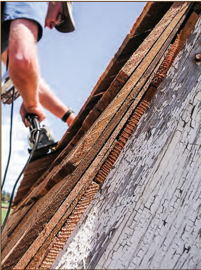
Figure 261—This edge view of the stud barn roof at the Nine Mile Ranger Station (Lolo National Forest, Northern Region) shows rakers and three layers of shingles. The shingles immediately above the fascia are rakers. You can tell which shingles are rakers because their end grain is exposed, rather than the edge grain exposed on the sides of other shingles.
