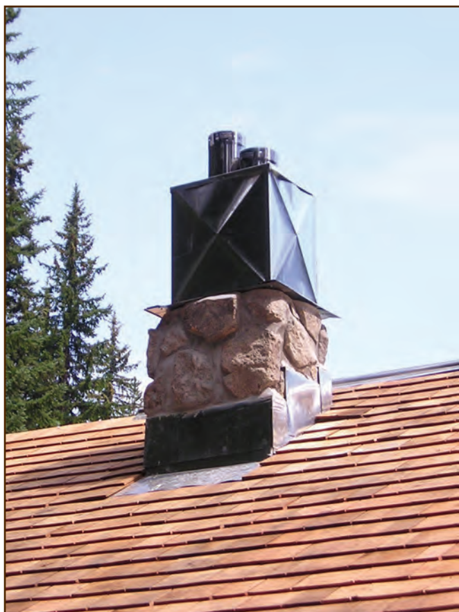
Figure 248—Preservation crewmembers replaced the flashing all around the chimney at the Lost Horse cabin (Bitterroot National Forest, Northern Region).
