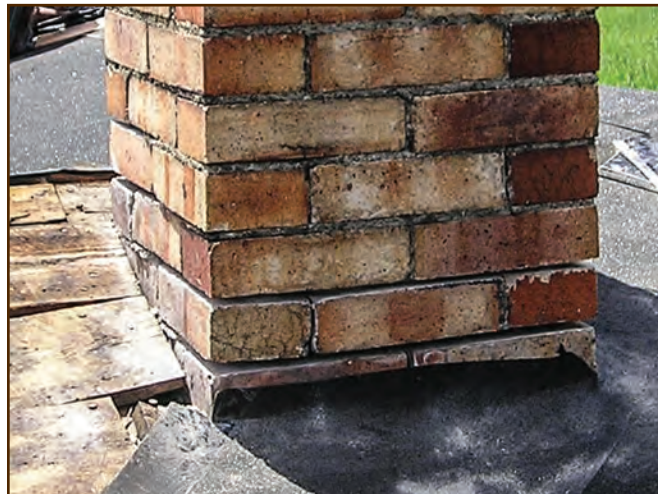
Figure 242—In preparation for reflashing, a preservation crewmember raked out the mortar from the joints on the chimney of the house at the Main Boulder Station (Gallatin National Forest, Northern Region) built in 1905.
