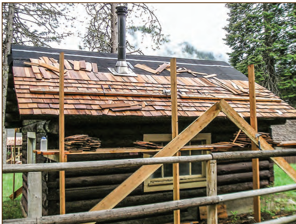
Figure 268—Roofers are installing a new shake roof on the Wash House at the Moose Creek Wilderness Station (Nez Perce National Forest, Northern Region). This 1937 log building has solid roof sheathing.
