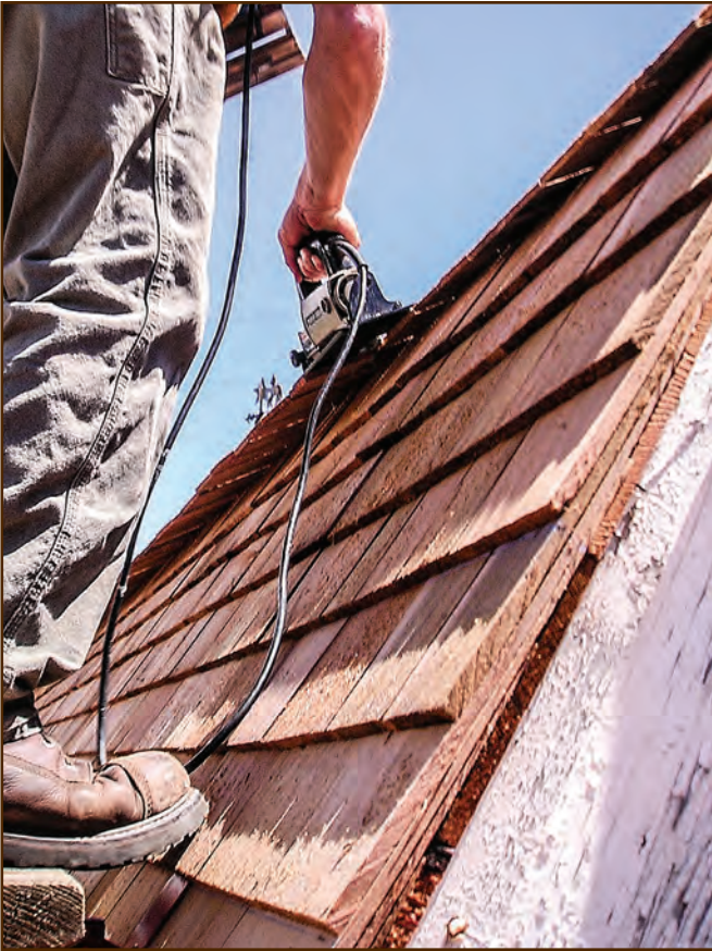
Figure 264—This roofer is using a small circular saw to cut off the first course of shingles on the gambrel of the stud barn at the Nine Mile Ranger Station (Lolo National Forest, Northern Region).
