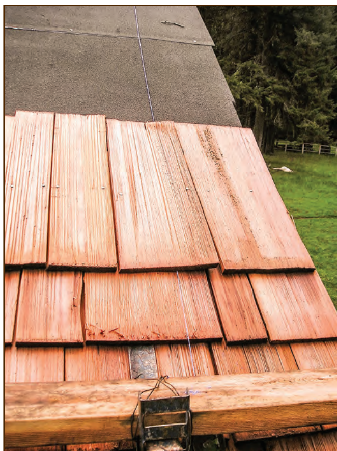
Figure 263—You can use a chalkline to produce even spacing for rake edge overhangs on both shingle and shake roofs. Roofers are installing this shake roof on the Office/Cookhouse building at the Moose Creek Wilderness Station (Nez Perce National Forest, Northern Region).
