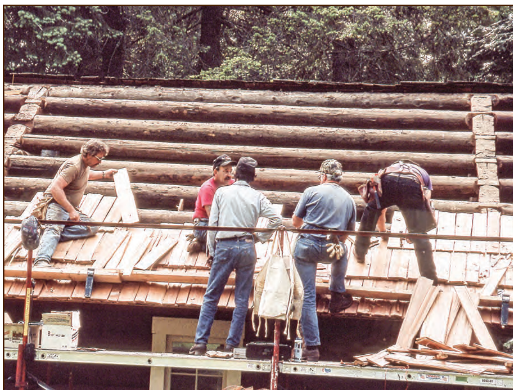
Figure 271—This crew laid 32-inch-long shakes on the purlin roof of the fire cache at the Moose Creek Wilderness Station (Nez Perce National Forest, Northern Region) during the 1990s. If they were laying the shakes today, they all would wear hard hats and would wear fall protection harnesses while working on the upper courses.
