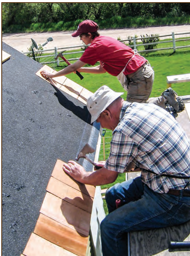
Figure 239—The roofer at the top of the photo is laying raker shingles. The other roofer is laying the starter course. Before laying any shingles, the crew covered the entire roof with ice and water shield underlayment.
