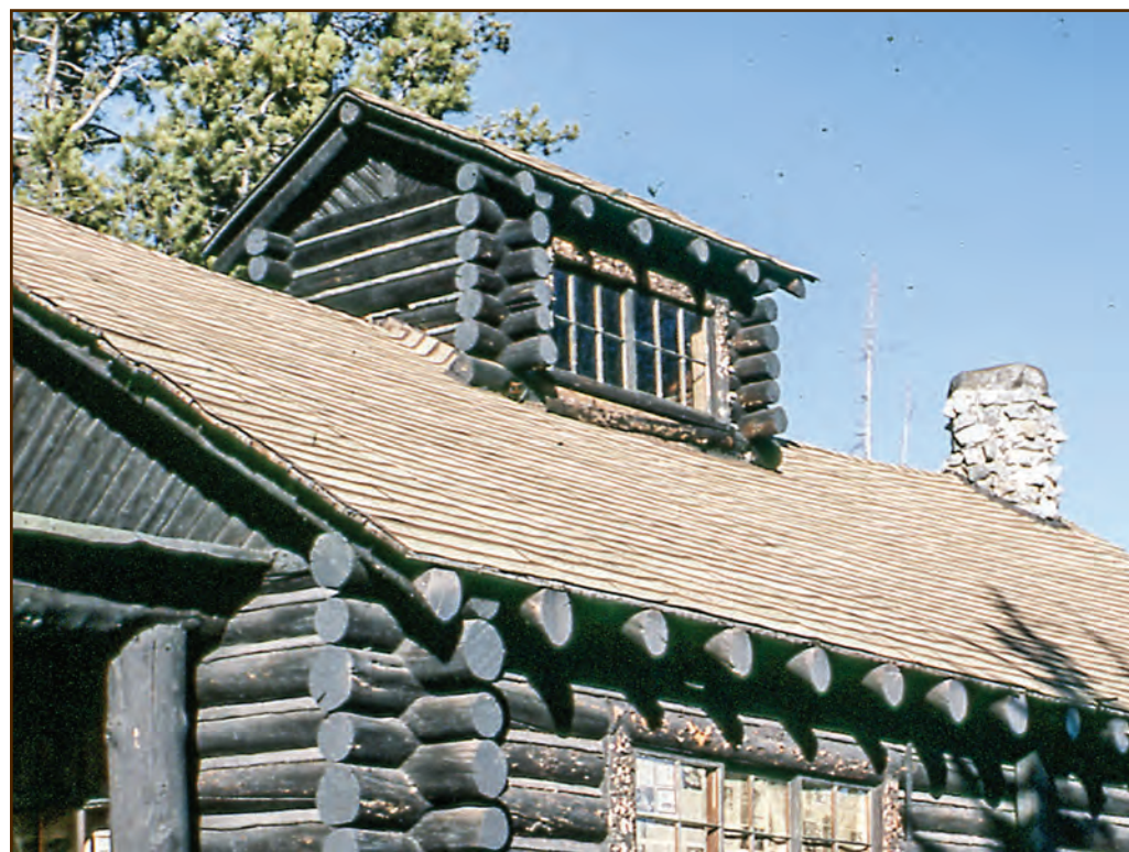
Figure 237—The builders placed a cant strip under the shingles that bend up the side of the cupola on this cabin in Grand Teton National Park in Wyoming.
