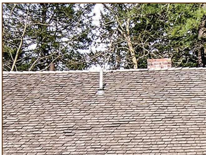
Figure 252—The shakes around this small vent in the Moose Creek Ranger's House (Nez Perce National Forest, Northern Region) required little trimming.
