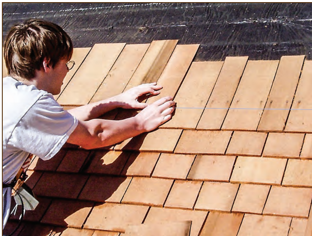
Figure 266—This roofer is laying shingles in courses on the west house at the historic Ninemile Ranger Station (Lolo National Forest, Northern Region). The shingle courses are evenly spaced due to careful measuring and the use of chalklines. The chalkline for the current course is visible in the photo. The horizontal spaces between the shingles are reasonably even.
