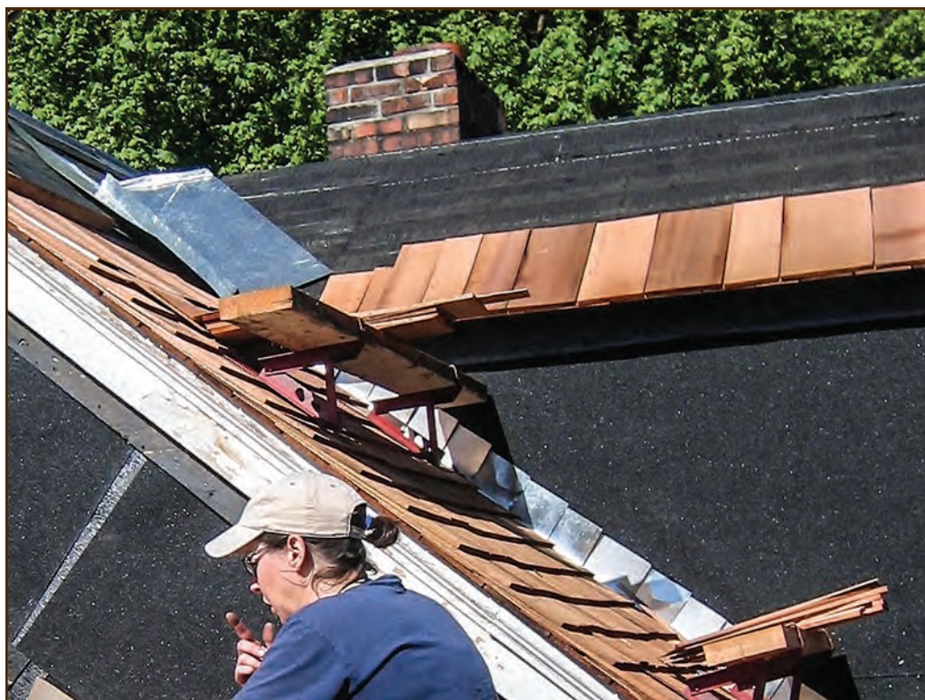
Figure 241—This roofer is installing galvanized steel step flashing and valley flashing during the reroofing of this complex roof at the historic Ninemile Ranger Station (Lolo National Forest, Northern Region).
