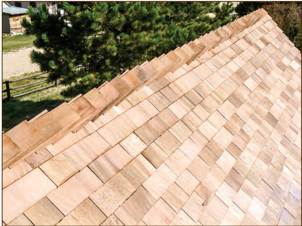
Figure 275—Preservation crewmembers constructed this shingle ridge cap when they replaced the roofing at the Ninemile Ranger Station (Lolo National Forest, Northern Region).
