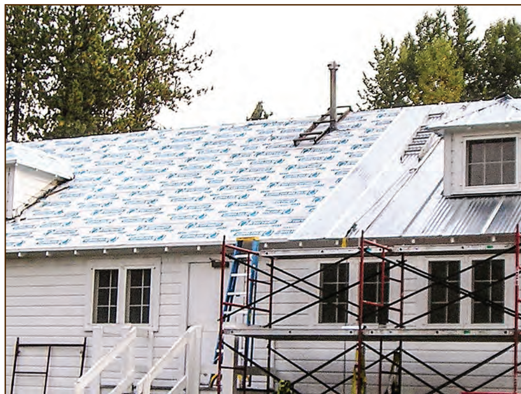
Figure 278—Preservation crewmembers are laying a new corrugated metal roof over ice and water shield on the Sav-enac Tree Nursery Bunkhouse (Lolo National Forest, Northern Region), built in 1930. The roof is the same kind you would find on log cabins of a similar vintage that have metal roofs.
