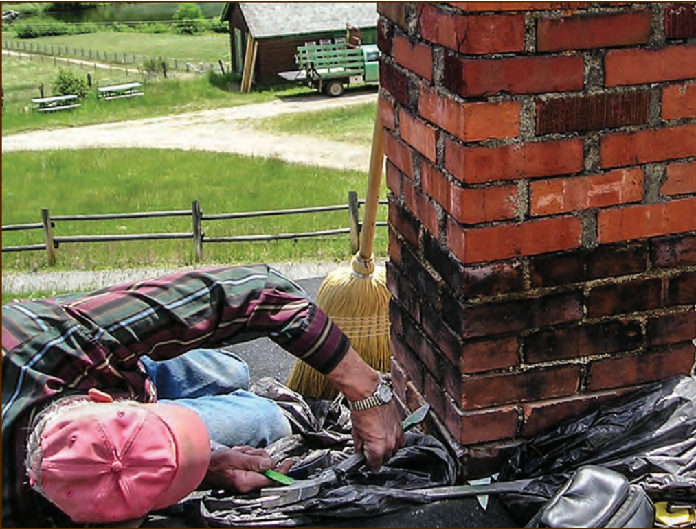
Figure 243—This preservation crewmember is using a hammer and plugging chisel to rake the joints on the chimney of a house built in 1905 at the Main Boulder Station (Gallatin National Forest, Northern Region).
