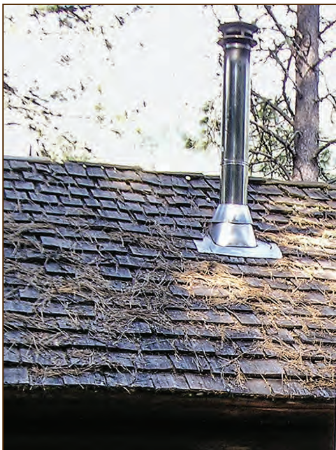
Figure 251—A preservation crewmember trimmed the shingles around this booted flue on the Moose Creek Wash House (Nez Perce National Forest, Northern Region).
