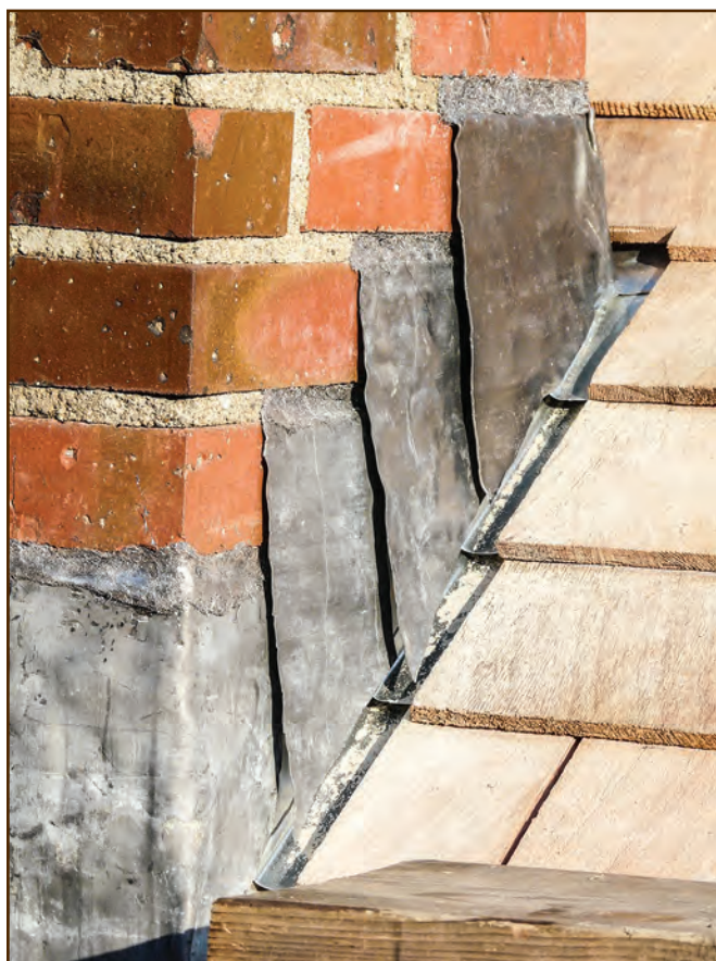
Figure 246—This closeup view of the chimney constructed in 1905 at the Zortman Guard Station within the Bureau of Land Management's HiLine District in Montana shows how the builder used lead sheets to counter flash the chimney. The builder stuffed lead wool into the masonry joints to match the original method of holding the counter flashing in place. The step flashing under the counter flashing is just barely visible.
