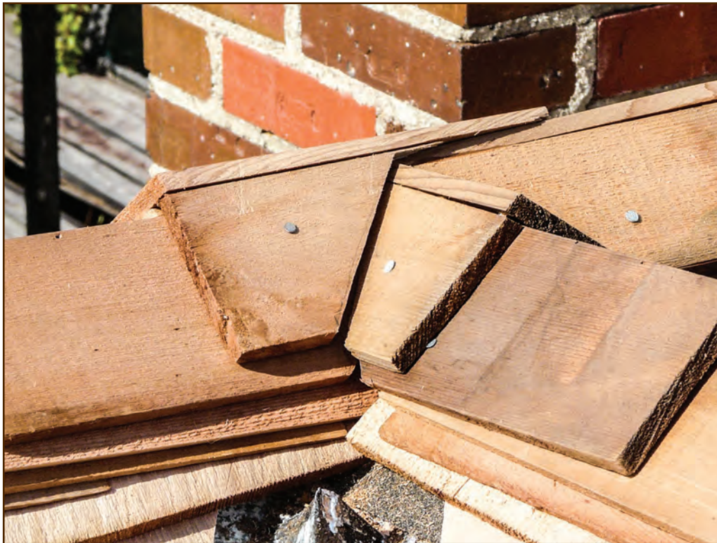
Figure 276—Preservation crewmembers constructed this complex shingle ridge cap while replacing roofing on the Zortman Guard Station within the Bureau of Land Management's HiLine District in Montana. The shingle butts switch direction in the middle of the roof peak, and a cross gable also intersects the main ridge line at that point. Because of the cross gable, the crew cut a notch into one side of the ridge cap unit at the middle of the roof.
