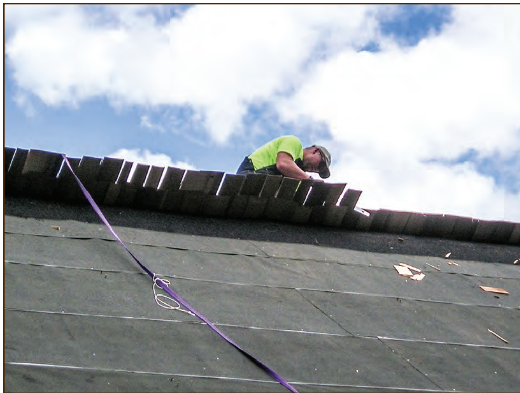
Figure 274—This roofer is using a small hand saw to trim the ends of the cock's comb ridge for the replacement roofing on the Moose Creek Wilderness Station Office/Cookhouse building (Nez Perce National Forest, Northern Region). Although the roof that the preservation crew replaced had a shingle ridge cap, historic photos showed that the original ridge cap was a cock's comb. The crew took the opportunity presented by the need for new roofing to restore the original configuration.
