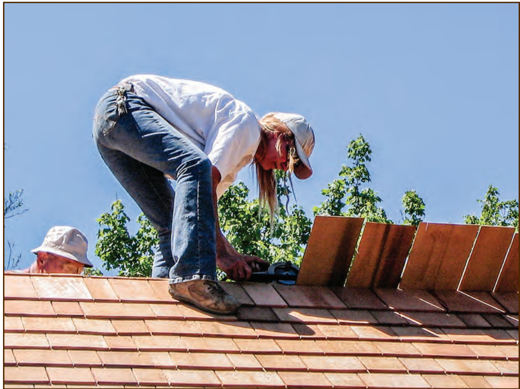
Figure 267—This roofer is using a small circular saw to cut the tails off shingles near the ridge of a roof.
