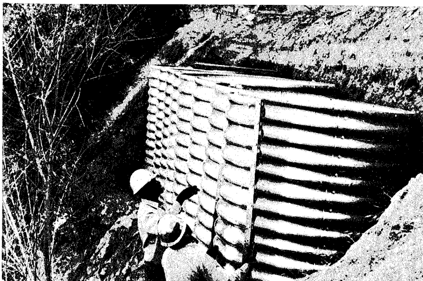
Figure 5. -- Positioning and bolting interstice facia sheets to bins.
