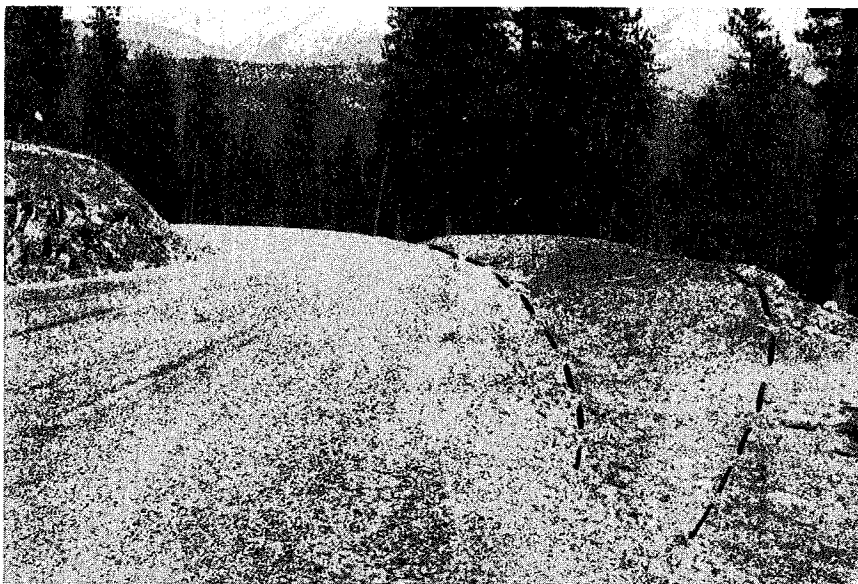
Figure 4. — New Road Prism
