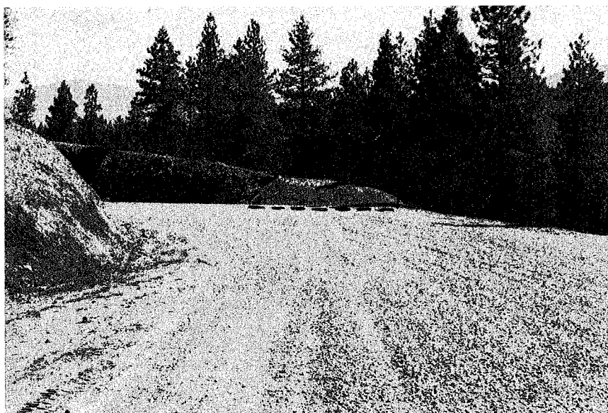
Figure 6. — Extension of a Cut Bank to Block the View of Old Roadbed
