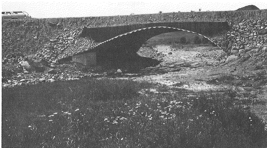
Figure 1. View of the 50 ft. x 10 ft. soil bridge from upstream in August 1975, after about 15 months of service.
