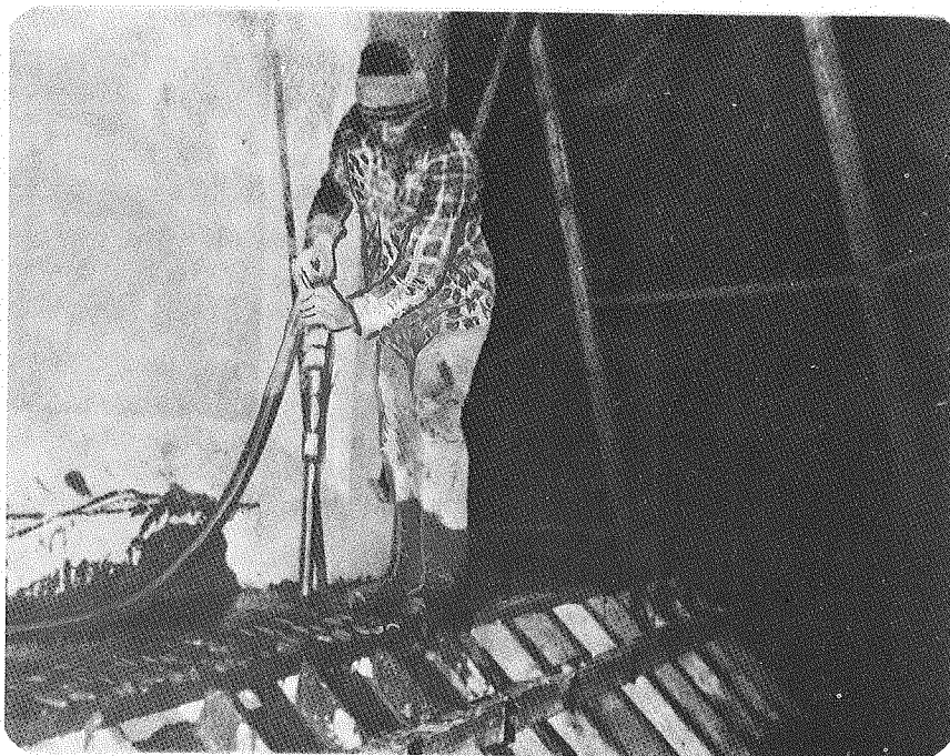
Figure 8. Final pumping of grout to eliminate air pockets.
