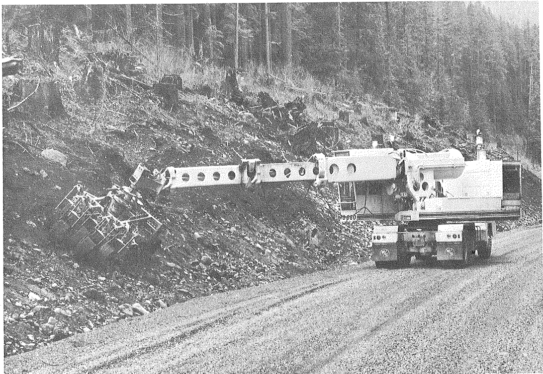
Figure 1.--SDEDC seeder, mounted on hydraulic telescoping boom machine, operating on littered cut bank on Willamette National Forest, Oreg.
