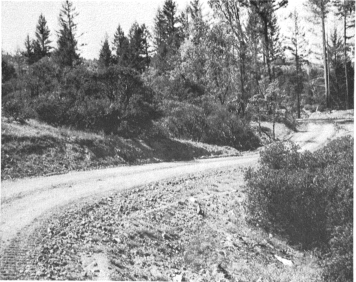
Figure 1.--Field-designed road, one season old; shows free-flowing grade and alignment, self-balance, and fill-and-cut sections.
