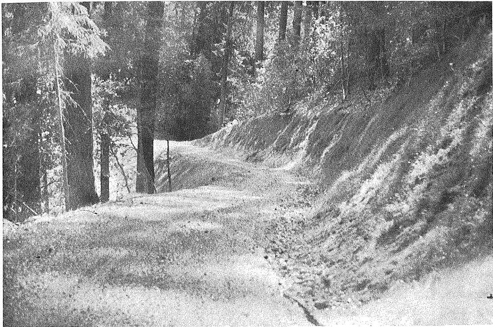
Figure 3.--Field-designed road on 60-75 percent sideslopes.
