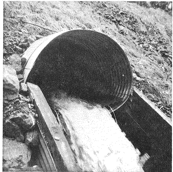
View showing the position of the replaceable corrugated metal liner at the outlet end of the pipe arch.
