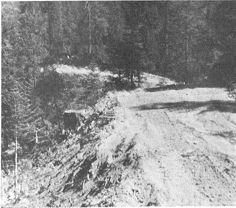
Figure 3.--Pioneered road with cleared side slopes.
