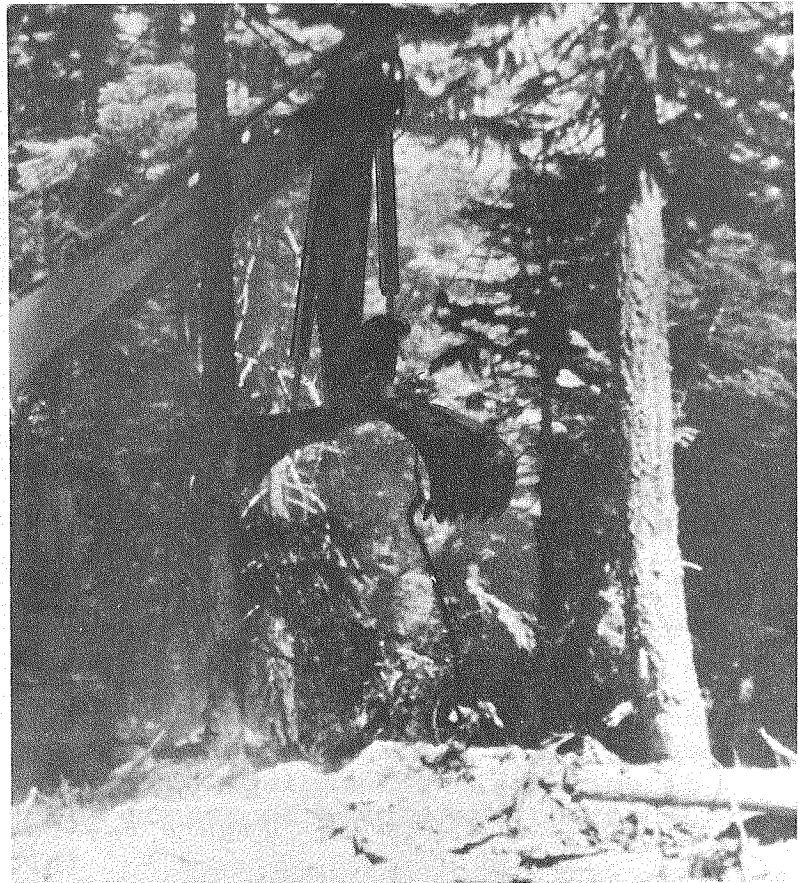
Figure 4.--Clam shell removing a tree.
