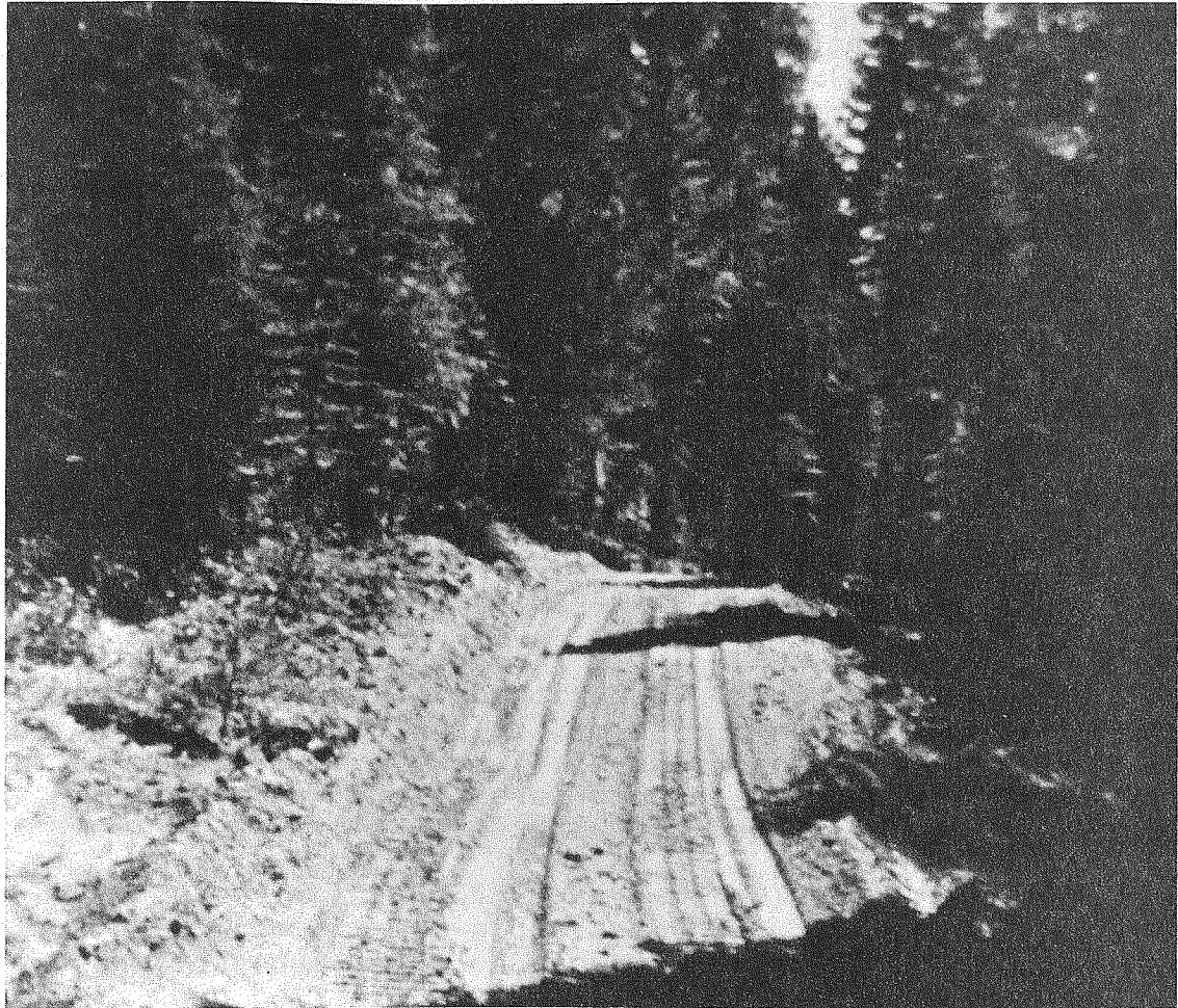
Figure 7.--Finished road, cleared by Model 225 with clam shell attachment.
