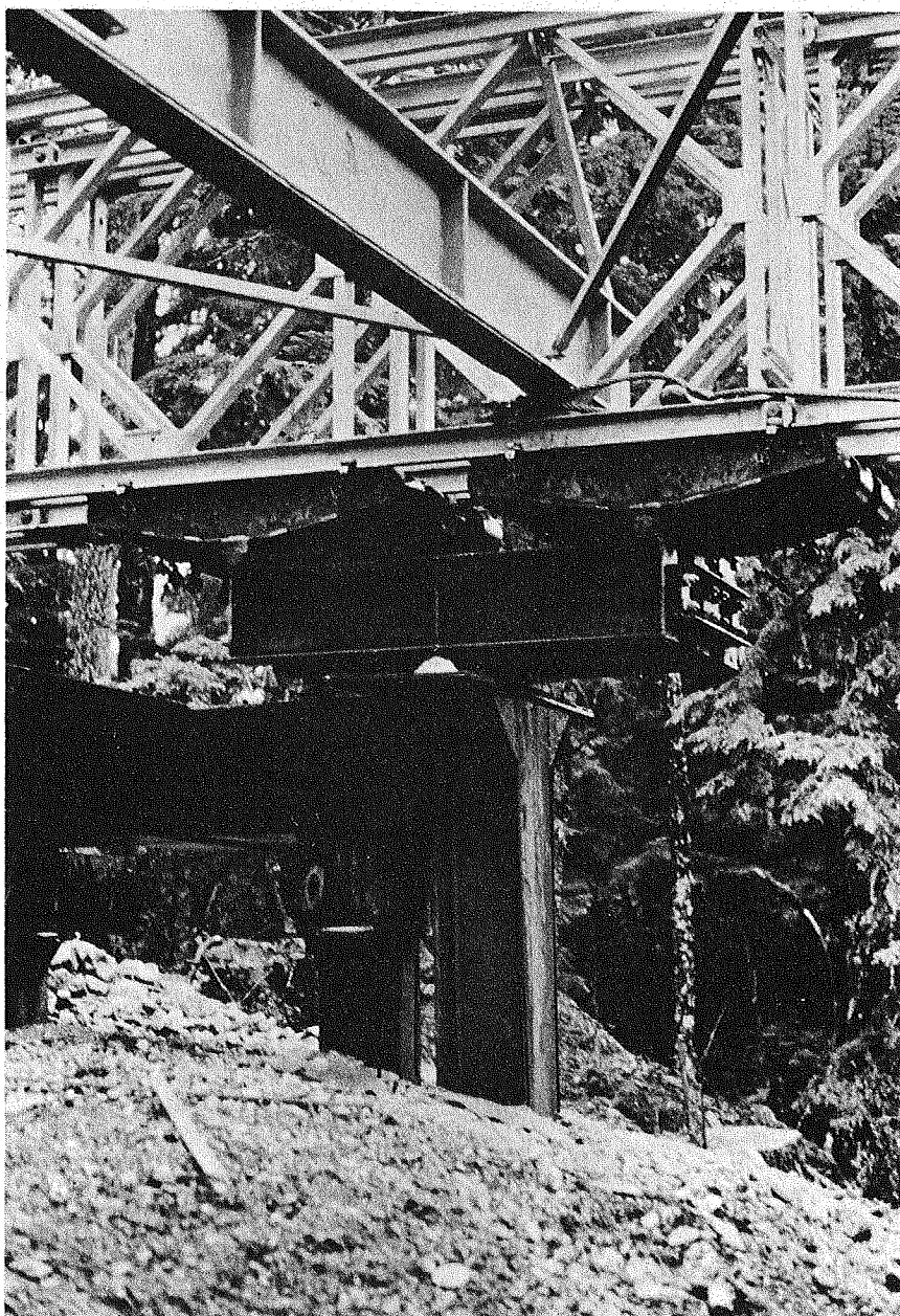
Figure 12.--Balance beam and rocking roller launching assembly. Entire weight of the bridge is balanced on these rollers just as the launching nose touches down on the far side.
