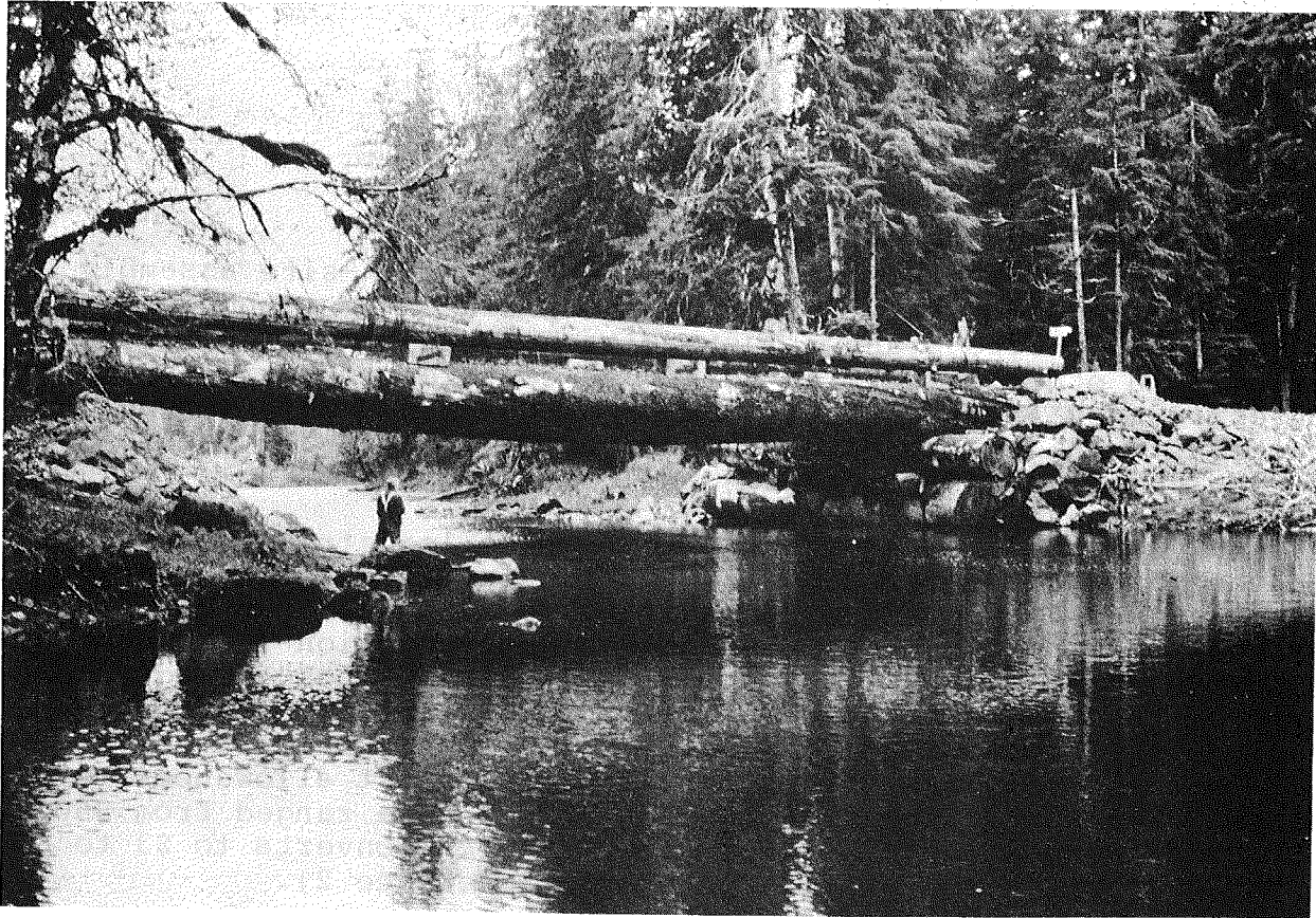
Figure 1.--Typical log stringer bridge.
