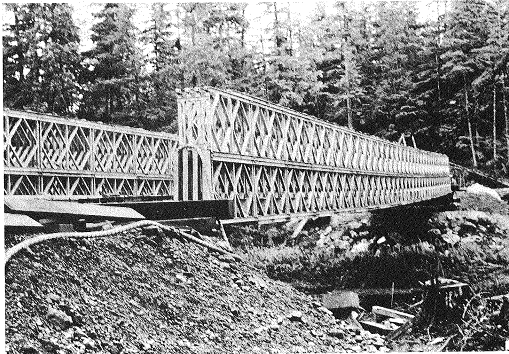
Figure 6.--Hamilton Creek Bridge--190-foot (57.91-meter) span Acrow Panel Bridge (quadruple-double reinforced construction).
