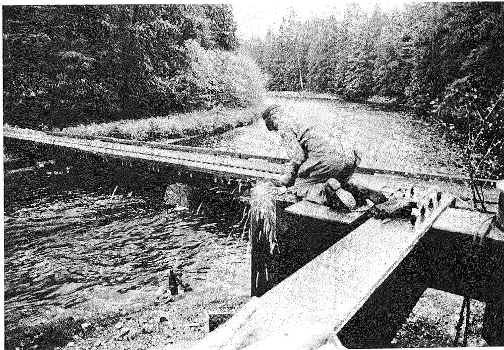
Figure 7.--Three Hamilton "E-Z" Bridges installed end-to-end as a temporary crossing during construction of the Hamilton Creek 190-foot (57.91-meter) Acrow Panel Bridge.
