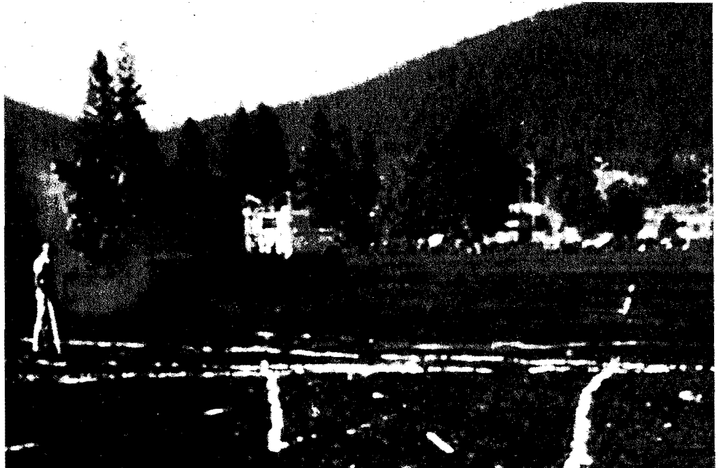
Figure 2.--Offtracking of the log truck as it leaves a curve on a tangent.
