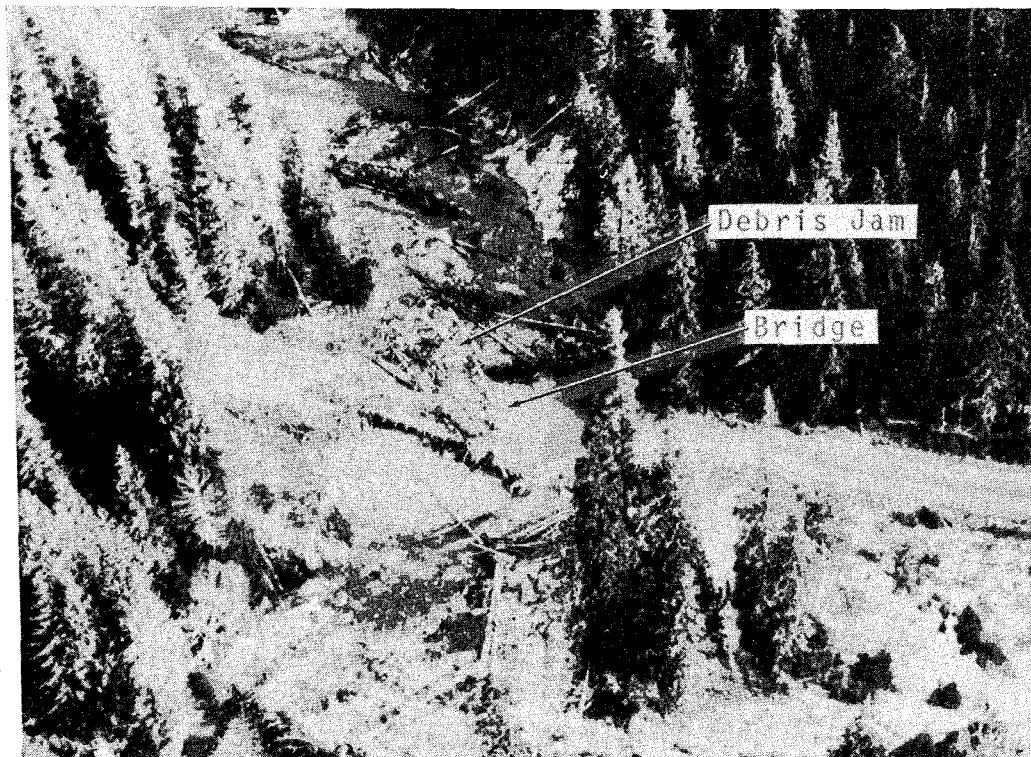
Figure 7.--East Fork Creek Bridge site.
