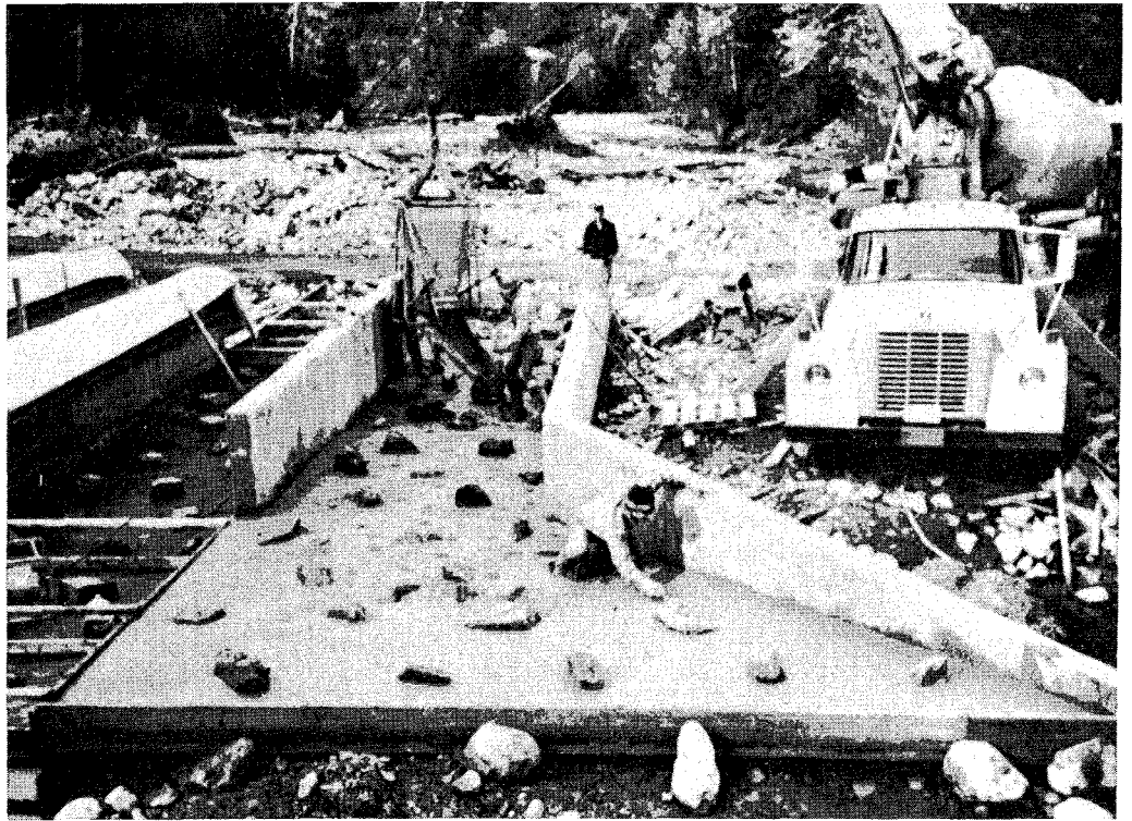
Figure 9.--East Fork Creek structure under construction.
