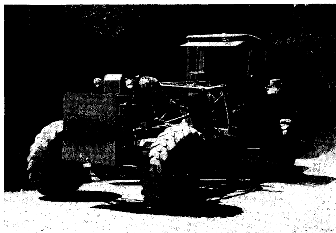
Figure 1.--About a quarter of the Forest Service's annual road budget goes to maintenance, such as this grading of an aggregate road on California's Six Rivers National Forest.
