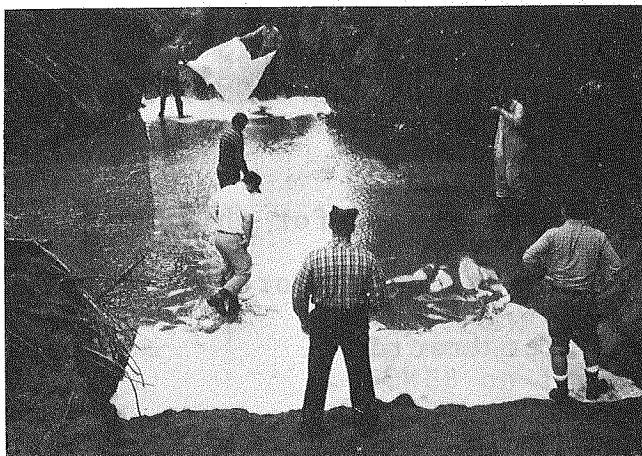
Figure 6.--Installing geotextile (Trivera 1127, nonwoven).
