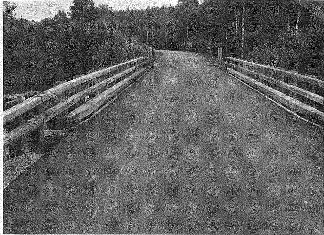
Figure 4.--Armstrong Creek Bridge after paving.
