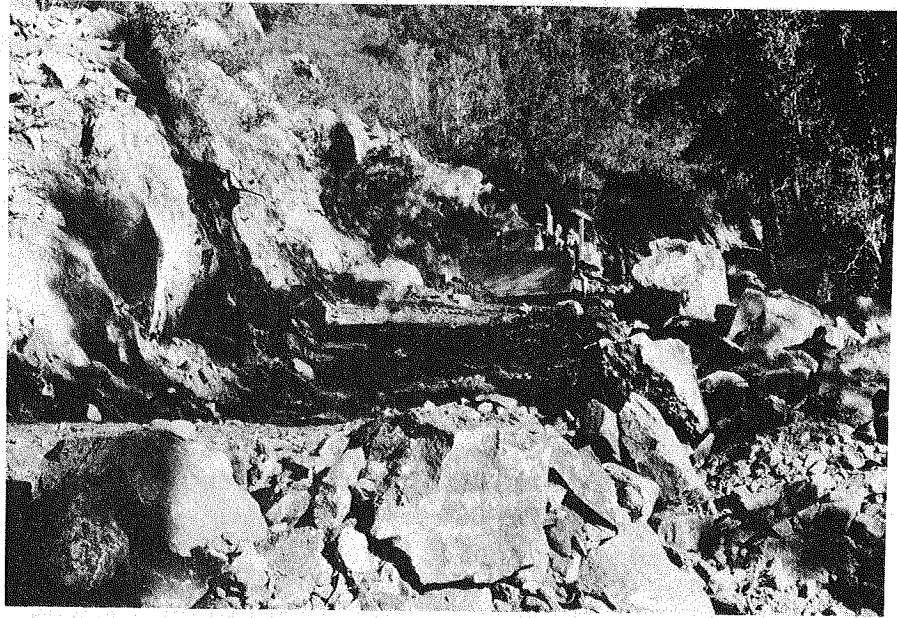
Figure 1.--Typical rock section during early stages of construction.
