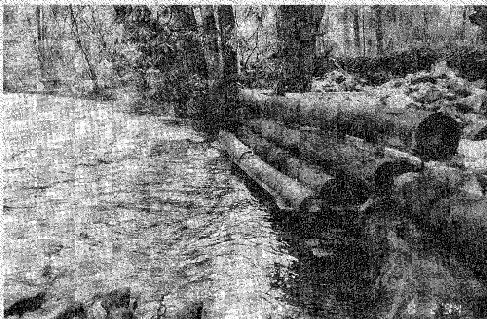
Figure 1.—Side view of 20-foot span structure showing trout cover.
