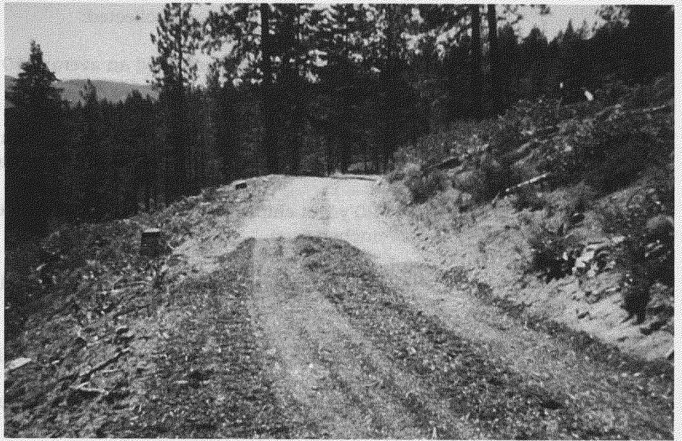
Figure 5.—Chips spread on the road.
