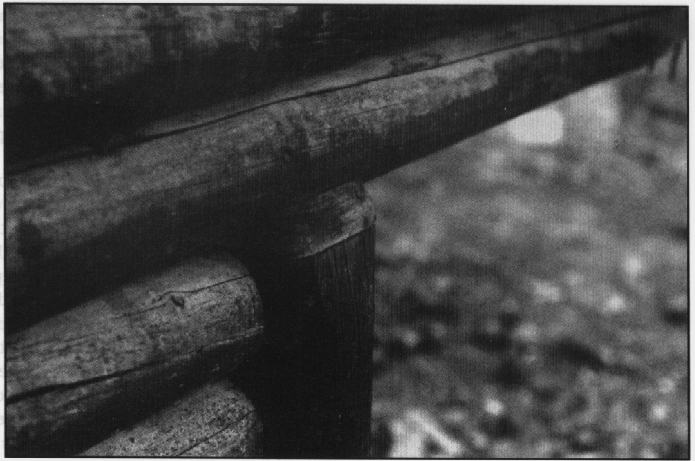
Figure 5. "Hog trough" corner-post system
