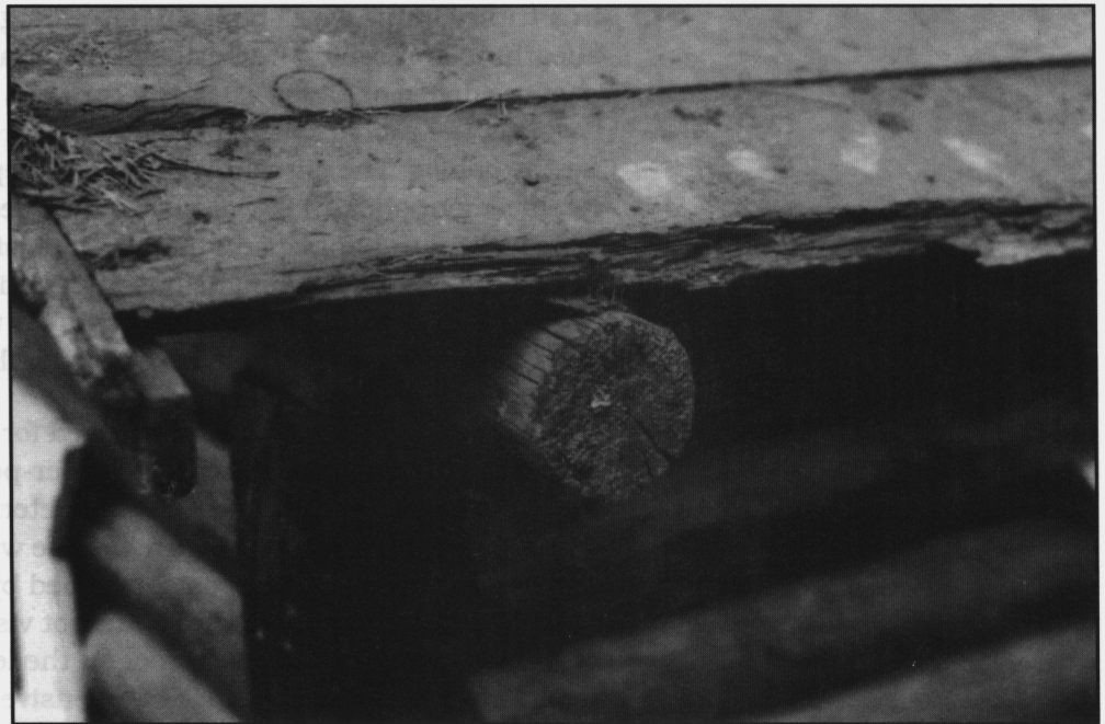
Figure 4. Missing shingles and broken shingles
