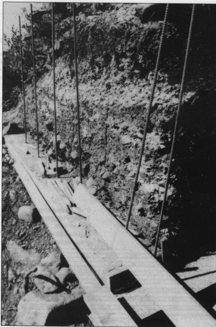
Figure 2. Concrete footing and vertical rebar constructed at base of prehistoric shell midden, is denoted by white shells and darkened soil behind rebar
