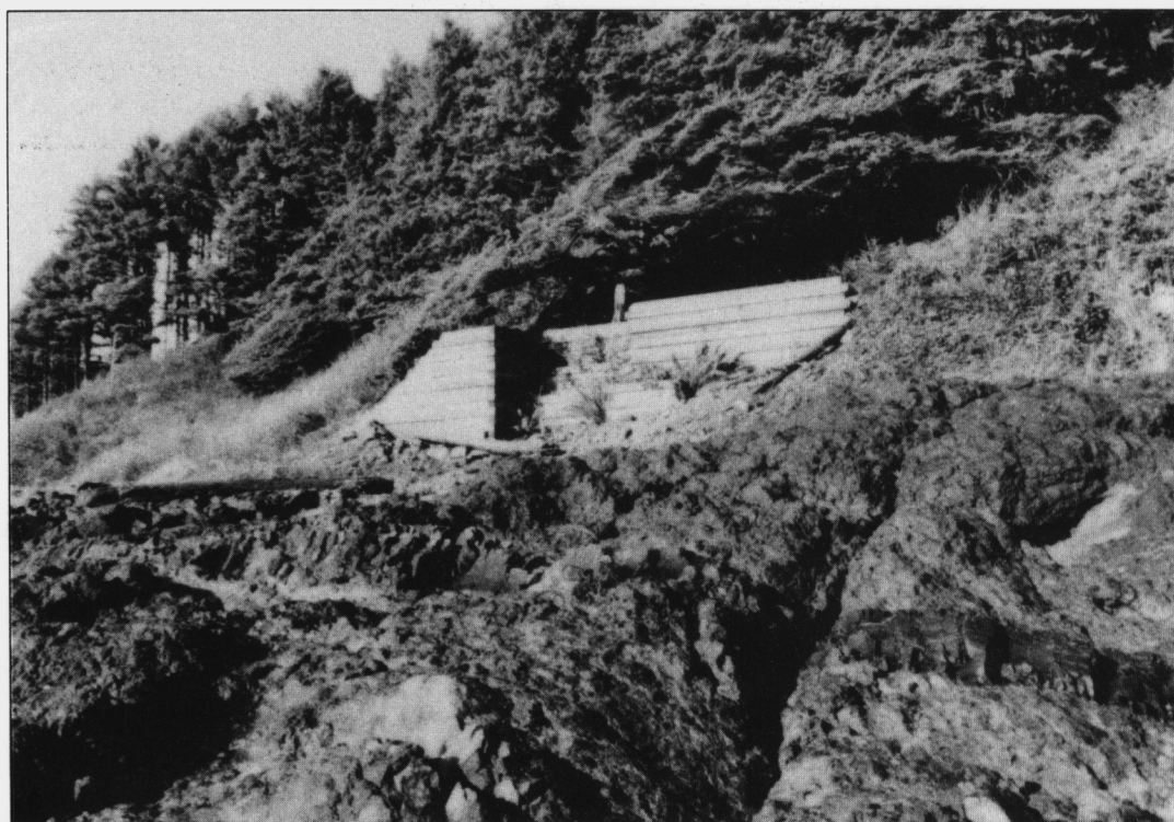
Figure 3. Completed sea wall at Cape Cove Shell Midden
